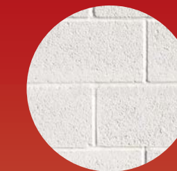
Original and Reclaimed CMU Blocks
