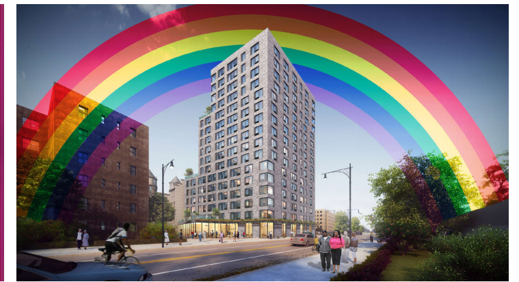
Fig. 25 The new Ingersoll Senior Residences apartment building
