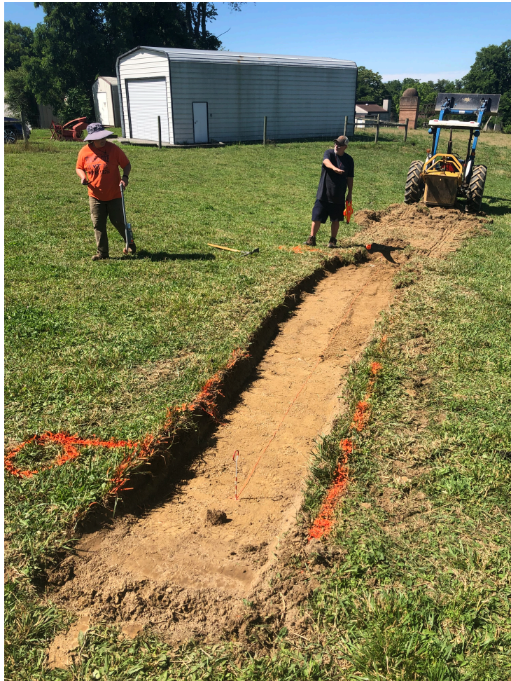
Figure 3.2. Ditch construction at PFRF using dirt scoop.
