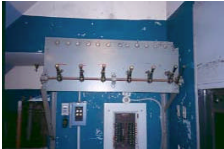
Figure 47. Light switches in projection booth, 2003.
