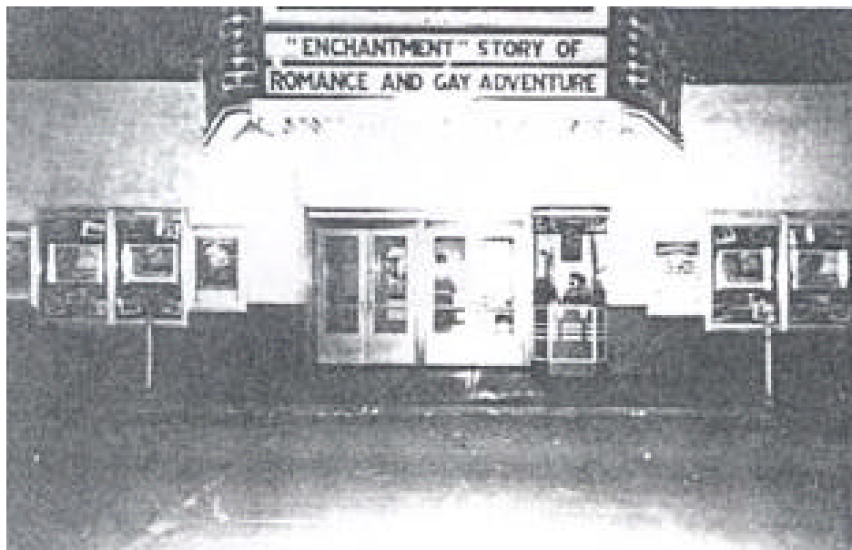
Figure 30. Ticket booth to right of doors, circa 1948.
