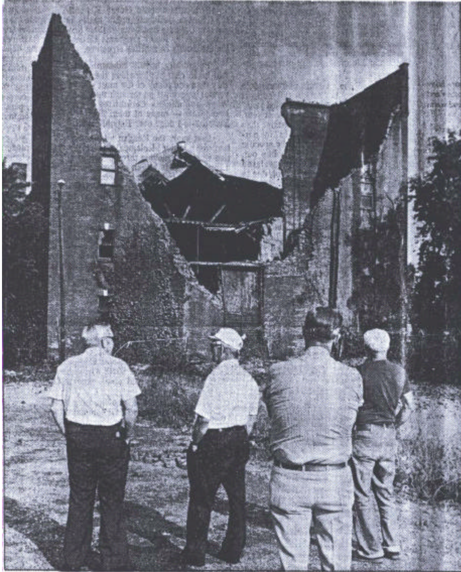
Figure 13. Dalton Theater collapse, June 12, 1982.
