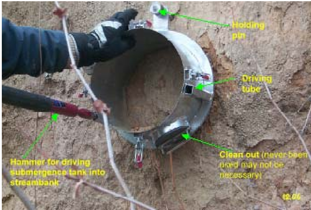
Figure G2. Placing submergence tank (picture courtesy of Dr. Greg Hanson, Research Hydraulic Engineer, USDA-ARS Hydraulics Engineering Research Unit, Stillwater, OK).
