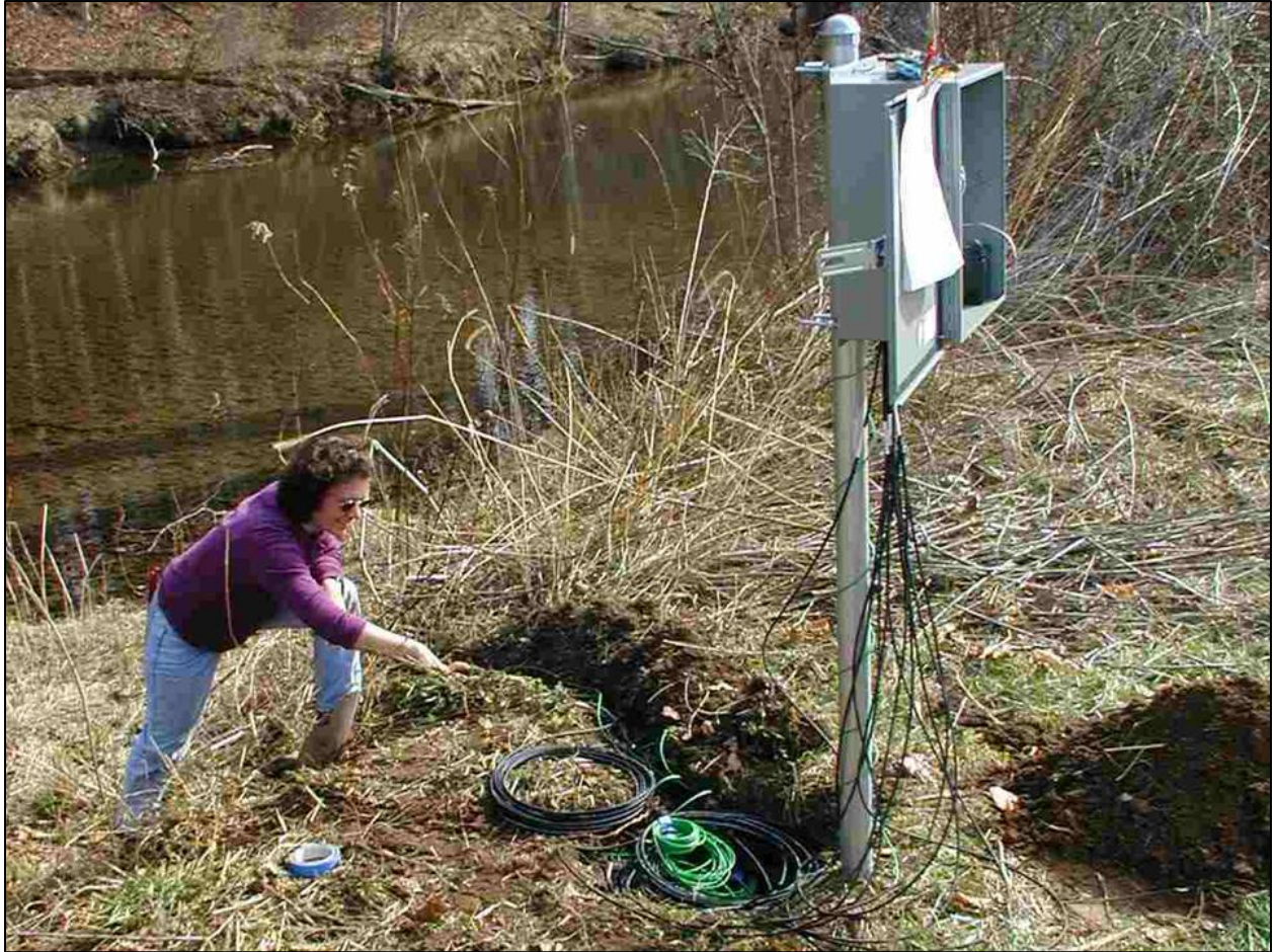
Figure 4.2. Installation of site SC6.
