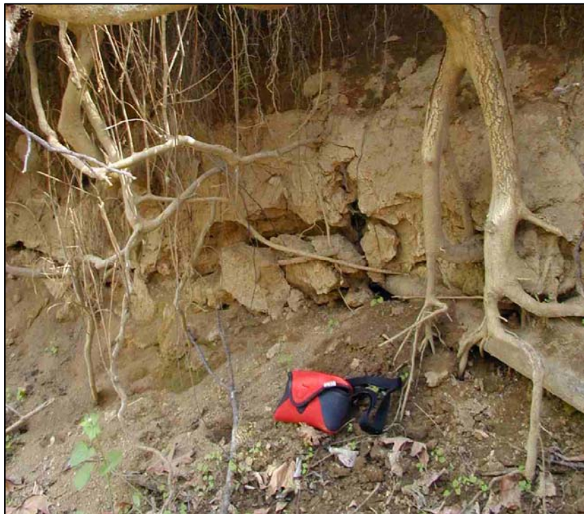
Figure 4.5. Stream bank degradation at site TC7 resulting from severe soil desiccation. Camera bag is approximately 18 cm in width.
