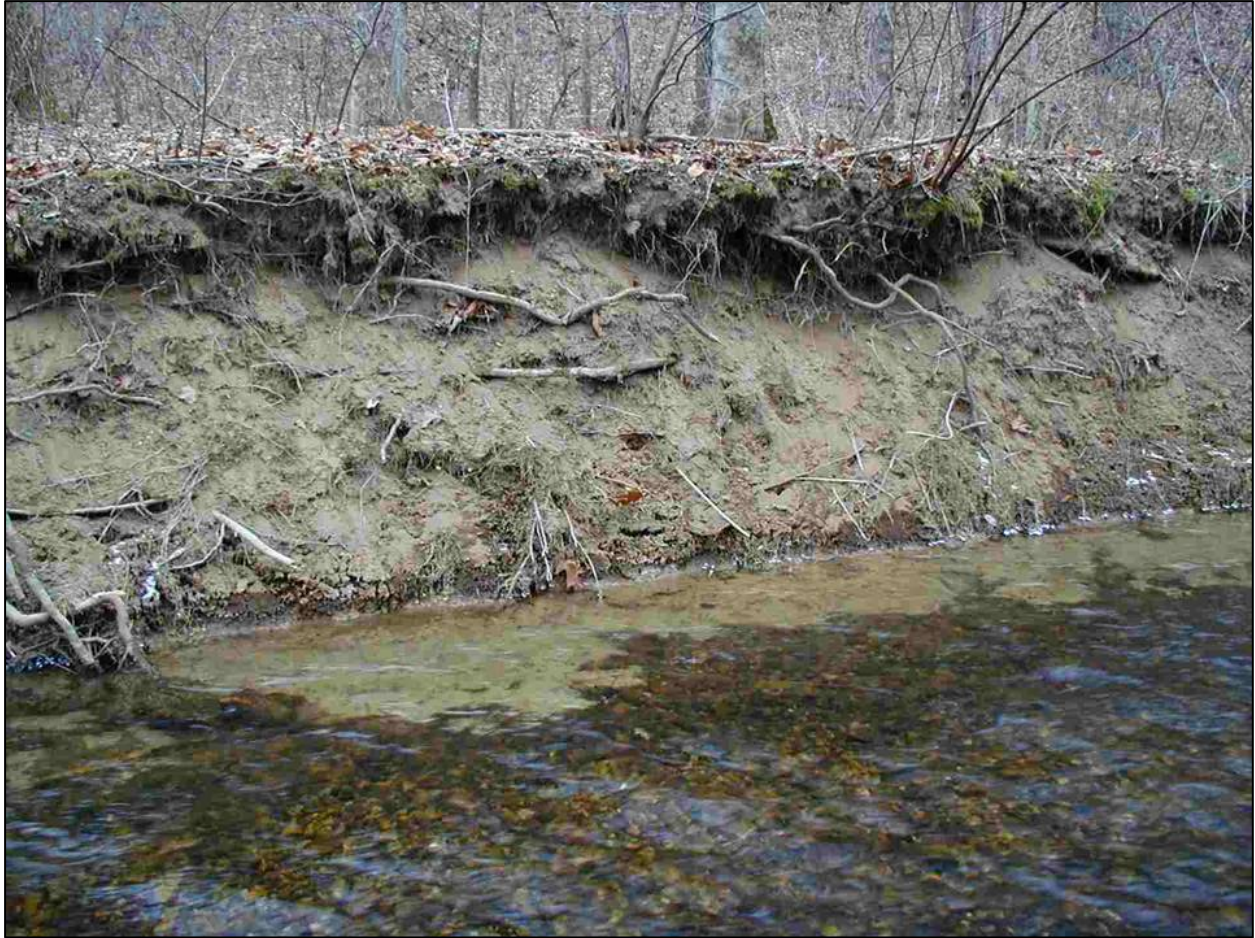
Figure 4.17. Loose soil on bank face of SC7 due to freeze-thaw cycling.
