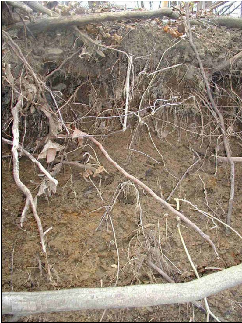
Figure 4.7. Loose soil at site TC4 resulting from freeze-thaw cycling.
