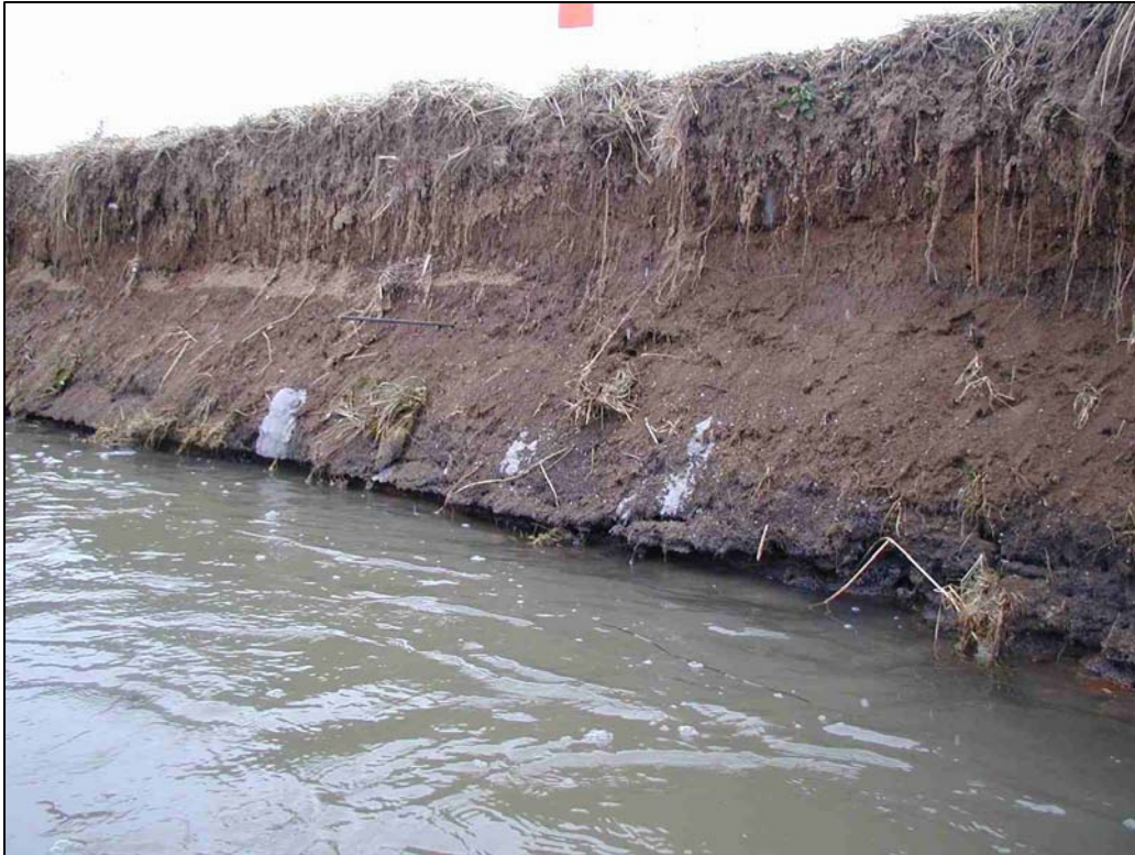
Figure 4.9. Erosional notch observed at site ST3.
