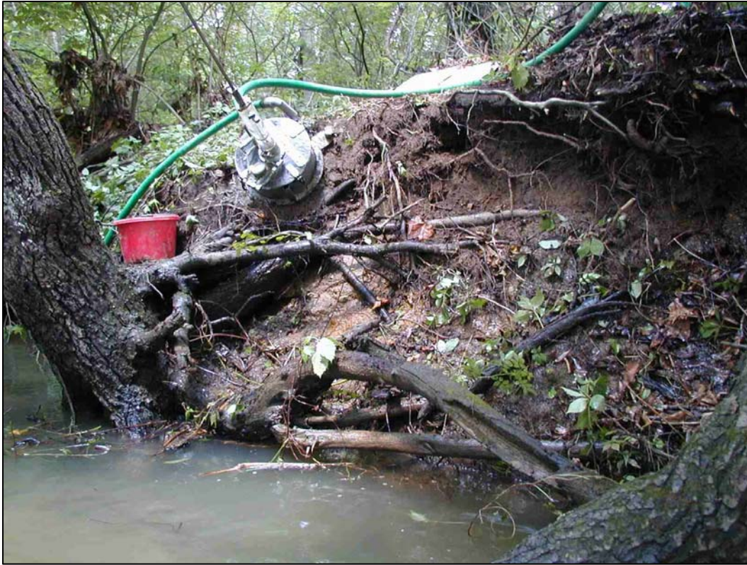
Figure 5.2. Jet test setup at heavily wooded site, TC4.
