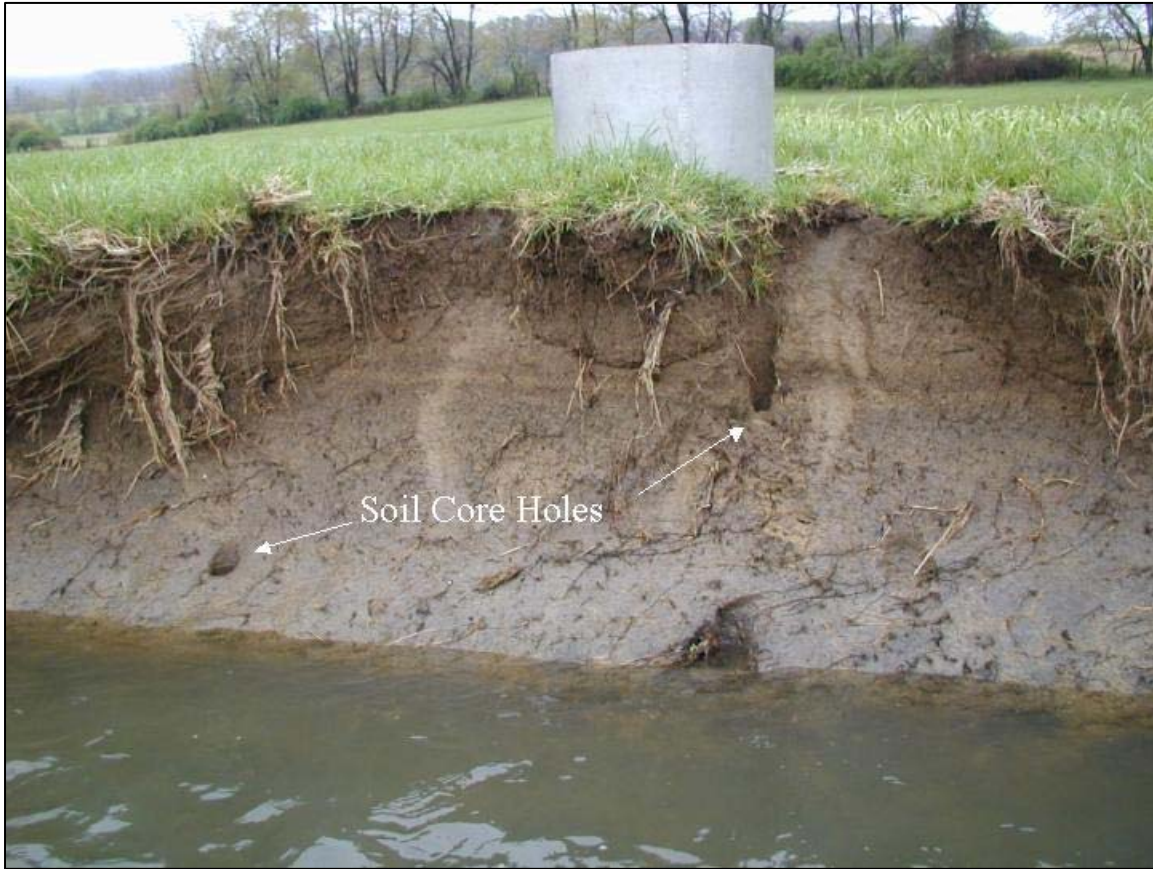
Figure 5.14. Soil core holes exposed at site ST3 during February 2003 flood. Bank exposure is approximately 1 m.
