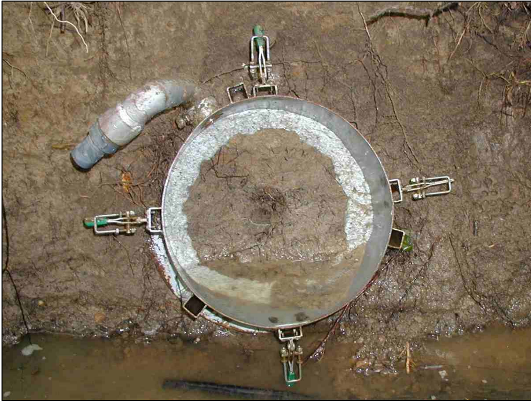
Figure 5.4. Bentonite seal around tank edge following test run.
