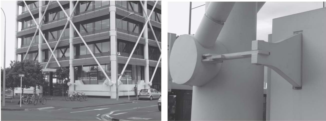
Figure 2.29 Triangular plate energy dissipating device (from Bruneau et al. 2011)
