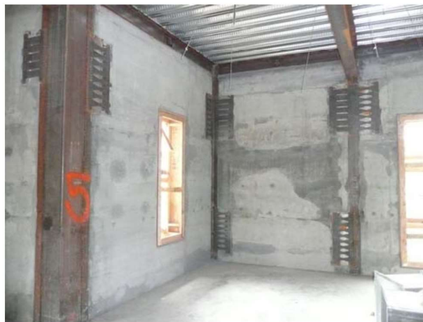
Figure 2.31 Fused Rotating Walls (Luth et al. 2008)
