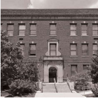
Figure 2.43 Safe Shores used to be Bundy School. The building has a history of helping people, including at one time housing the homeless 42 . It has since been renovated to accommodate office and therapy spaces for abused children in the DC area to advocate for child victims.
