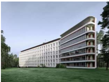
Figure 4.01 98 Paimio Sanatorium exterior photo
