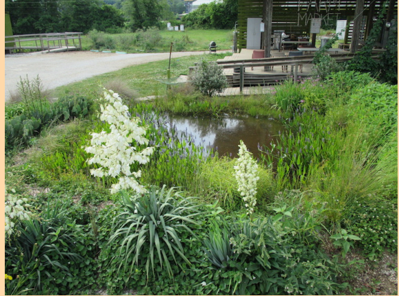
Figure 17-8: Turkey Nest pond after construction. The pond serves to capture rainfall and prevent erosion from an overflowing cistern.
