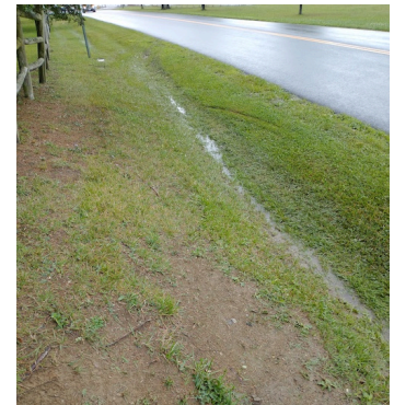
Figure 17-9: Swales capture water and move it from point A to point B.
