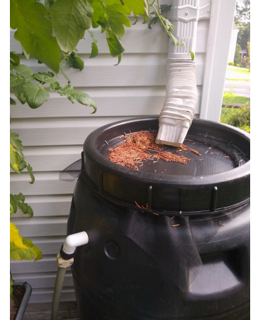
Figure 17-7: Rain barrel fed directly by downspout with overflow hose.
