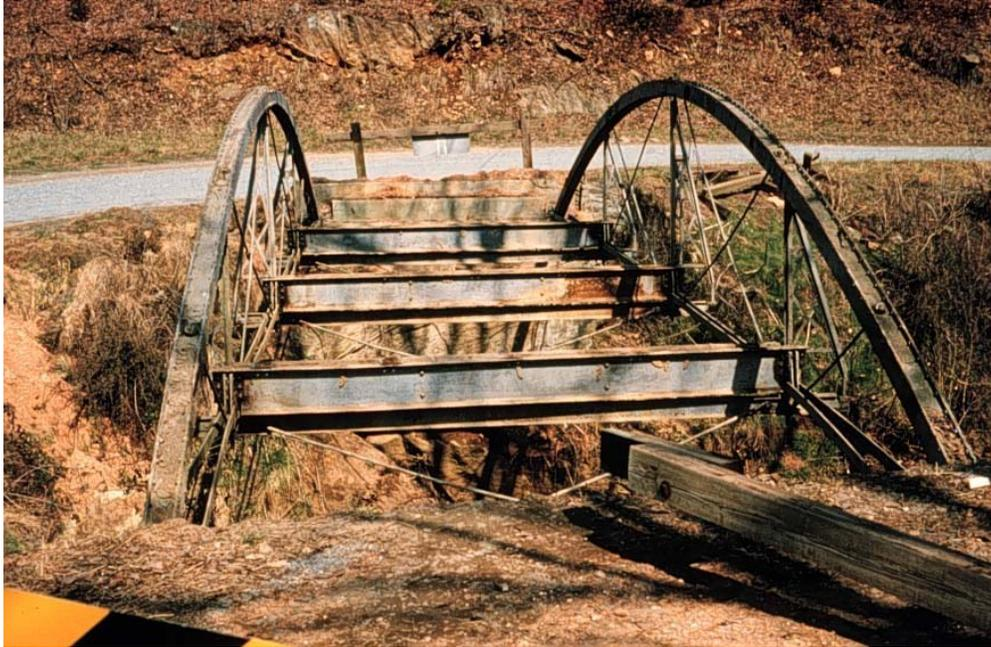
Figure 2 The bridge in Bedford County, VA with flooring system removed
