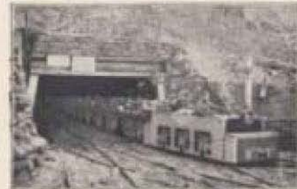
Electric Locomotive for Hoisting Purposes.
