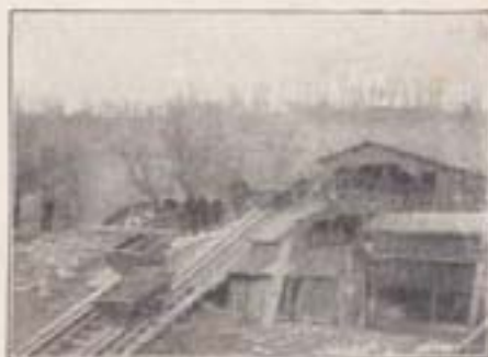
CHAIN AND WIRE CABLE CAR HAULS OF JEFFREY DESIGN OPERATE ON ALL GRADES
