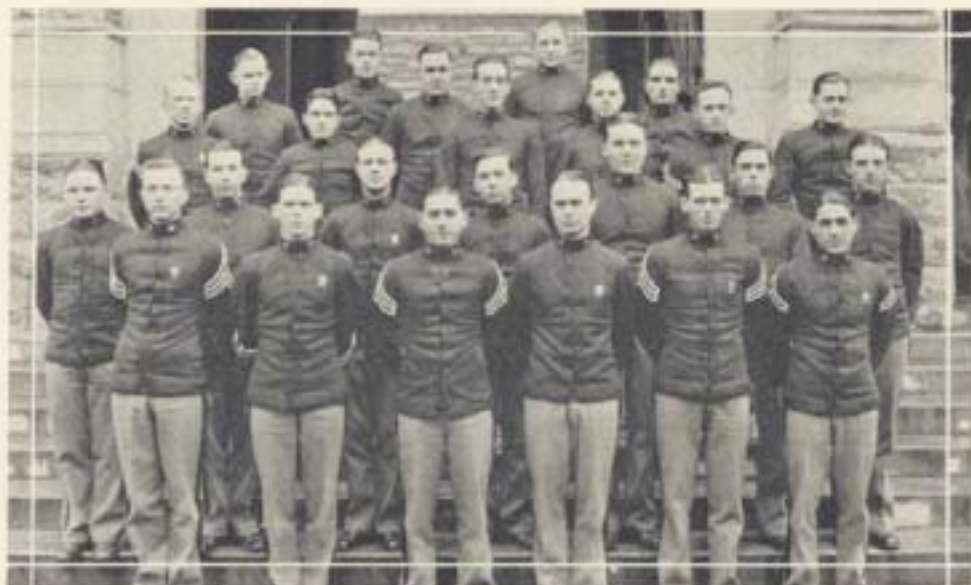
Three Hundred Sixty-Eight
