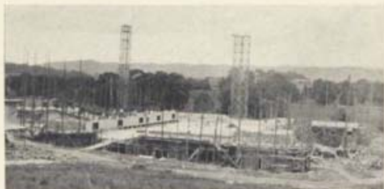
WAR MEMORIAL HALL FOUR MONTHS AFTER GROUND WAS BROKEN July 11, 1925
