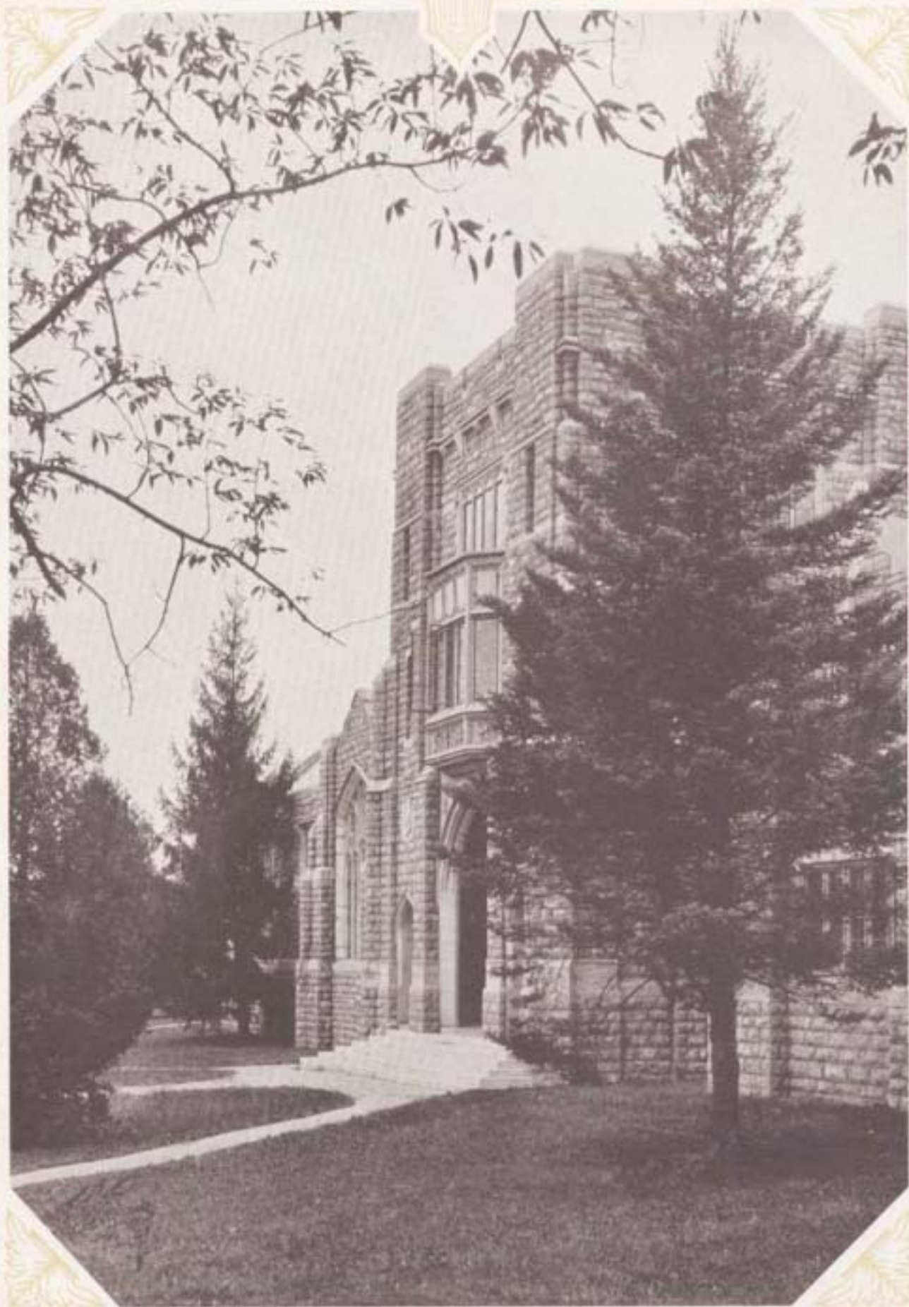
MAC BRYDE BUILDING "Each shafted ariel glimmers white"
