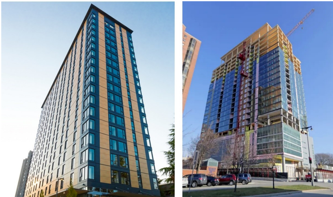
Figure 3. Mass timber buildings. Brock Commons Tallwood House in Vancouver, BC (18-storey, Left), Ascent in Milwaukee, WI (25-storey, Right)
