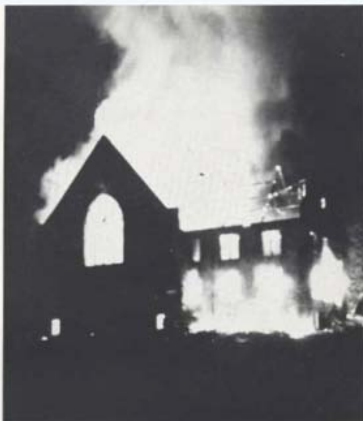
Demolished library, burned—1953
