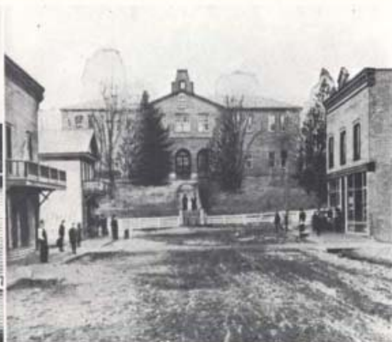
The Preston and Olin Building in 1907 shows the alterations which turned it into shops in 1889.
