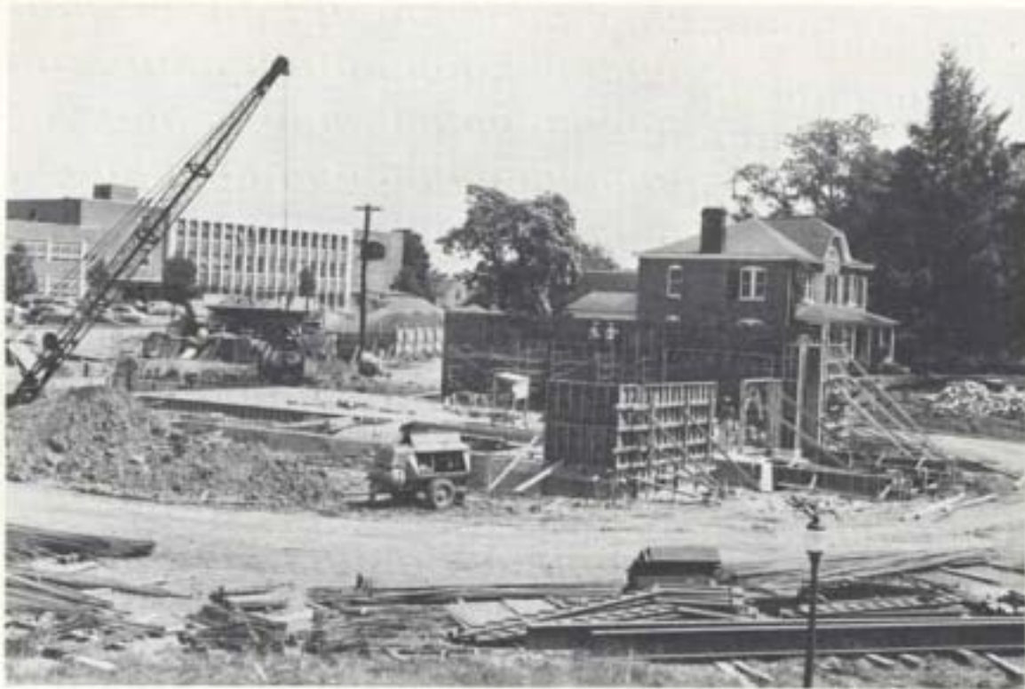
New Engineering Building construction.
