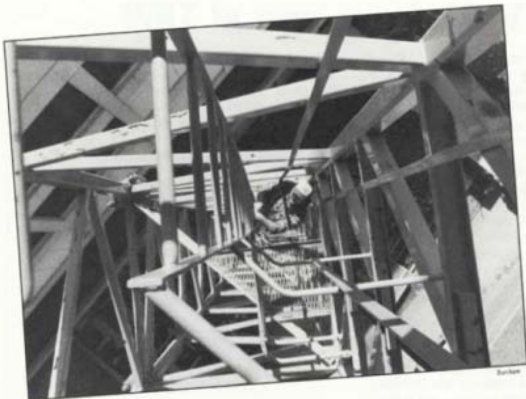
CLIMBING UP THE 150-foot vertical ladder each morning, Clark Anders works on the construction site to add additional floors to Whittemore Hall.
