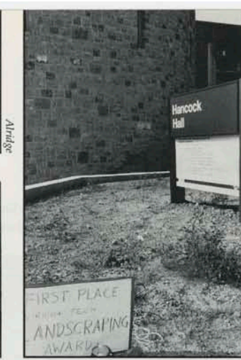
Hancock Hall, engineering building, completed in the fall
