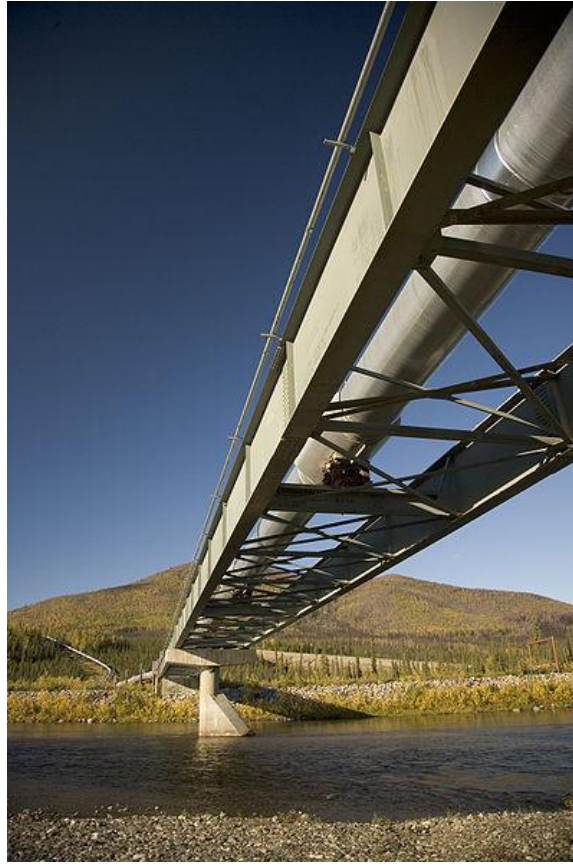
Figure 3 - This is a section of the Trans-Alaska oil pipeline crossing the South fork Koyukuk River [Public Domain].
