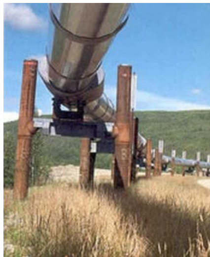
Figure 2 - Shown is an elevated section of the Trans-Alaska Pipeline. [Public Domain]
