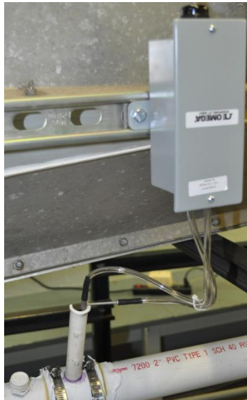
Figure 8. Pitot tube and differential pressure transducer
