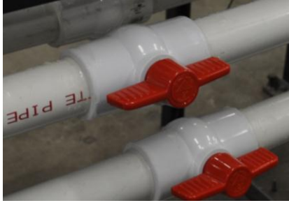
Figure 7. Valves used to simulate ventilation controls and mine airway damage
