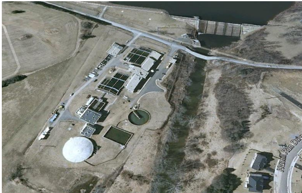
Figure 2-2 Aerial View of Lake Manassas Water Treatment Plant (August 2010)
