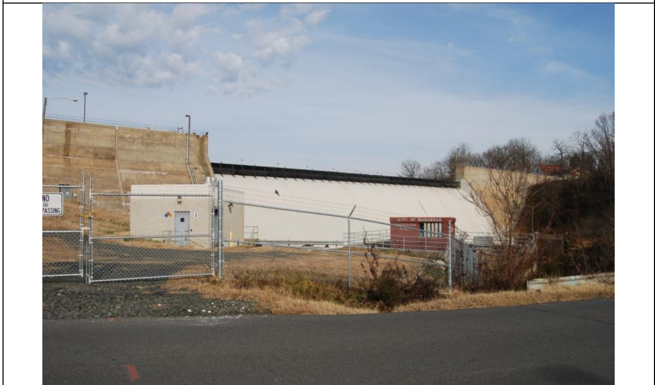
Figure A-6: T. Nelson Elliott Dam at Glenkirk Road showing rubber bladder on top – Facing North (NOV-2012)
