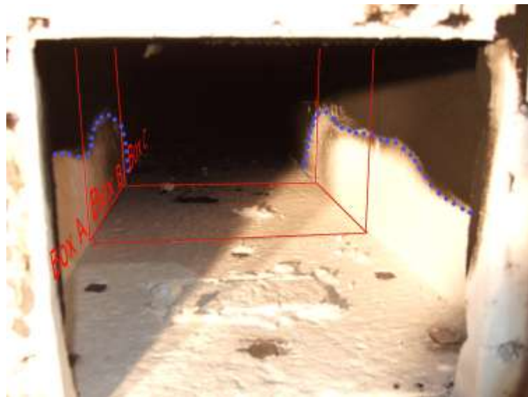
Figure 40. Post fire investigation of soot/flame patterns. Red lines indicate borders of cubic construction elements, blue dotted line indicates flame locations in the last part of the test (no soot patterns due to oxidation in flames)
