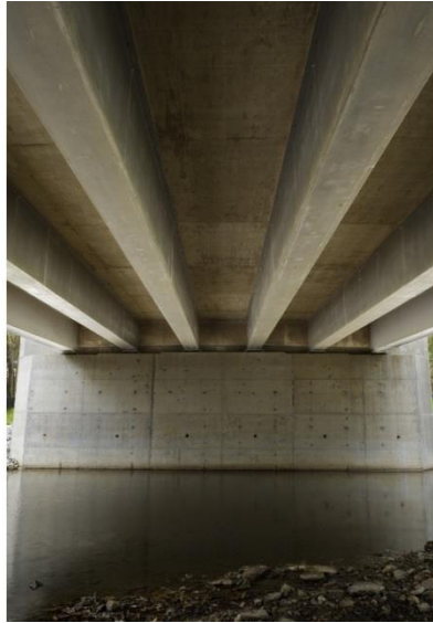
Figure 3-2 Underside of High Road Bridge in Illinois (from http://www.hcbridge.com )
