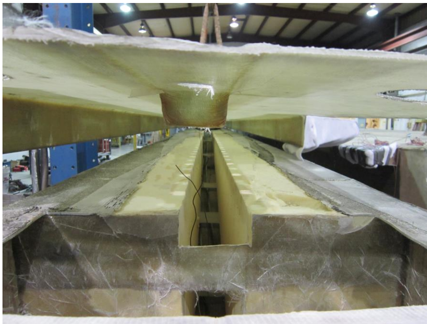
Figure 1-6 Placement of Lid onto FRP Shell
