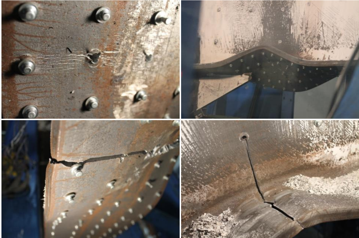
Figure 56: Test 12 - Initial PAF hole tearing (top left), Crack propagation (top right), Full flange fracture (bottom left), Fracture extension to web PAF hole (bottom right)
