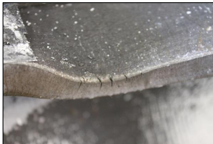
Figure 59: Tearing of the Flange Edge from Test 5
