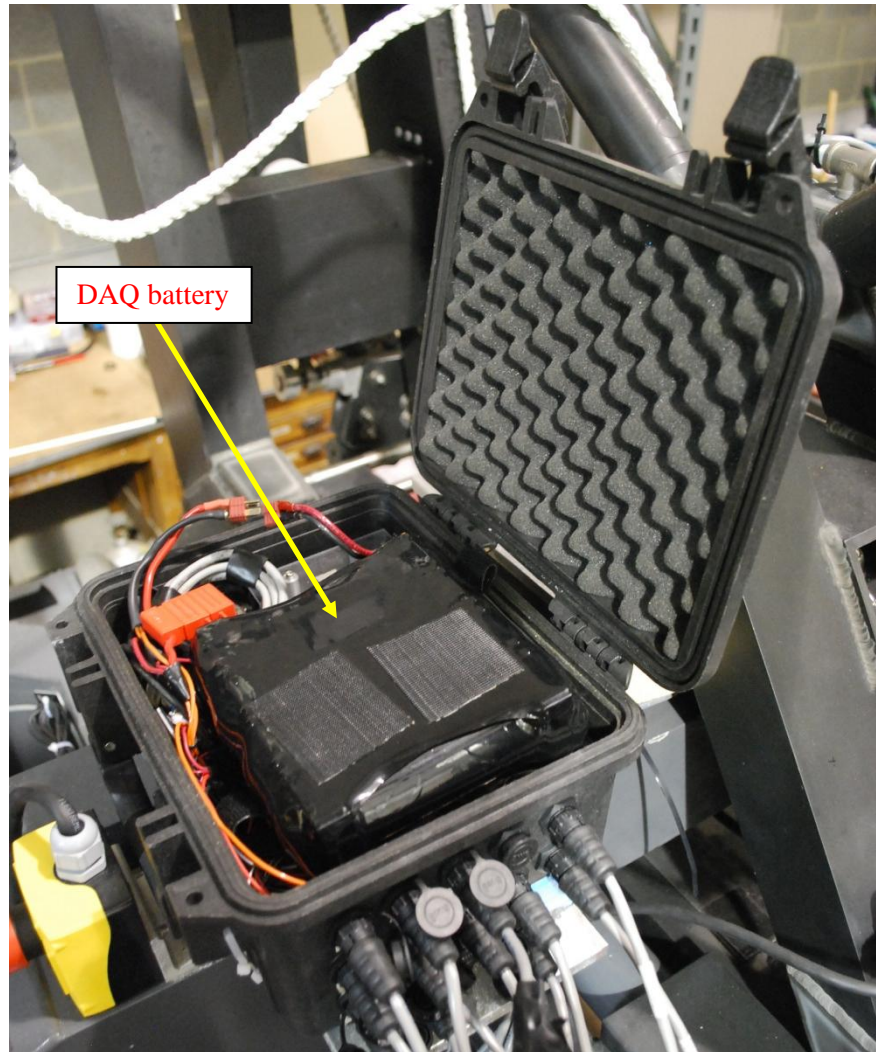
Figure 4-23: DAQ box containing cRIO, tri-axial accelerometer, and DAQ battery
