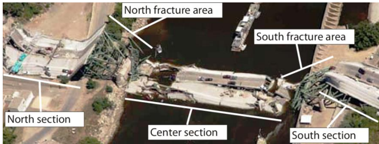
Figure 2.2-2: Collapsed deck truss north, center, and south sections of the bridge (Source: NTSB)
