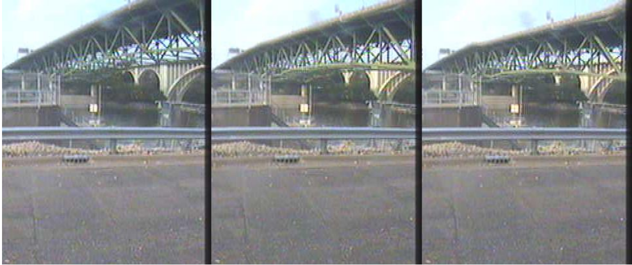
Figure 3.4-1: First three frames captured by the security camera during the collapse
