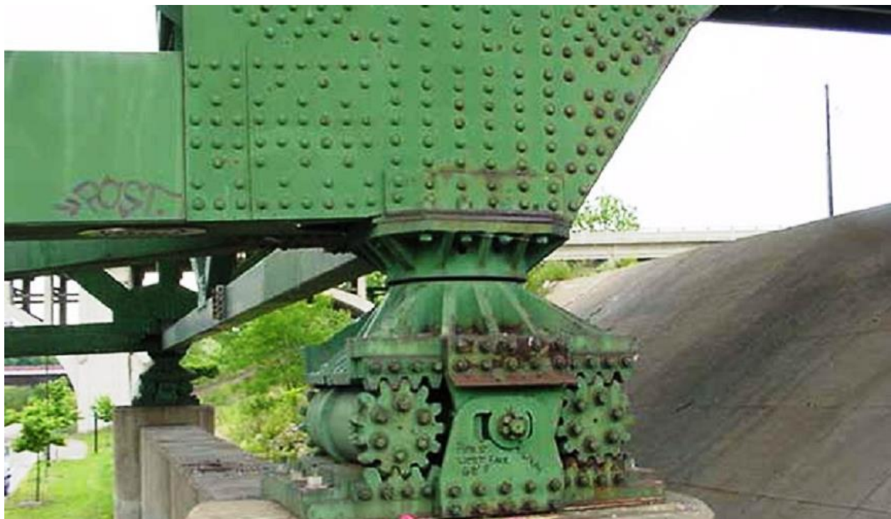
Figure 2.1-3: Expansion roller bearings at pier 5, looking east (Source: NTSB)
