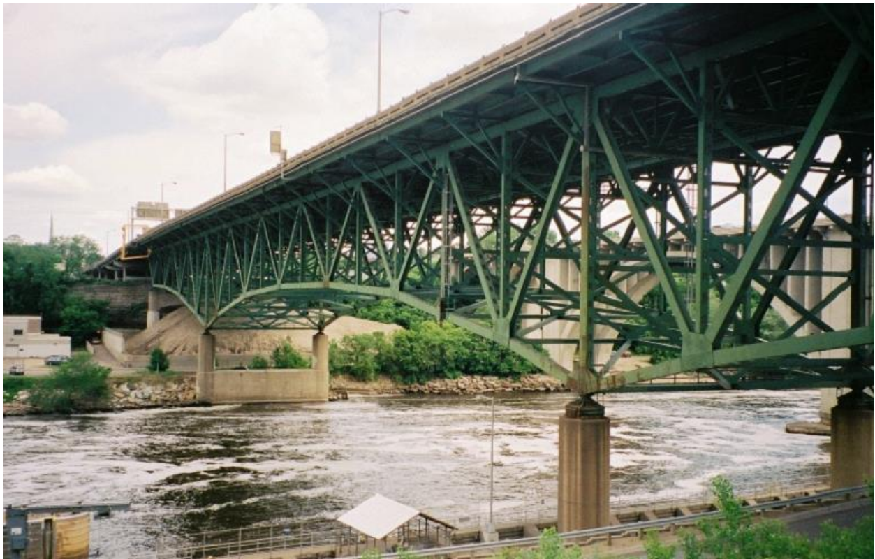
Figure 1.1-1: View of the deck truss portion of the bridge, looking northeast (Source: NTSB)
