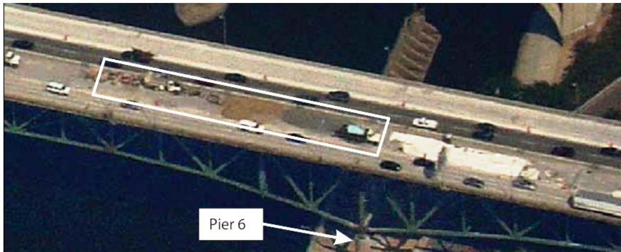
Figure 2.2-1: Construction equipment and aggregates about 2:15 hours before the collapse. (Enlargement of photograph taken by a passenger in a commercial airliner. Source: NTSB)
