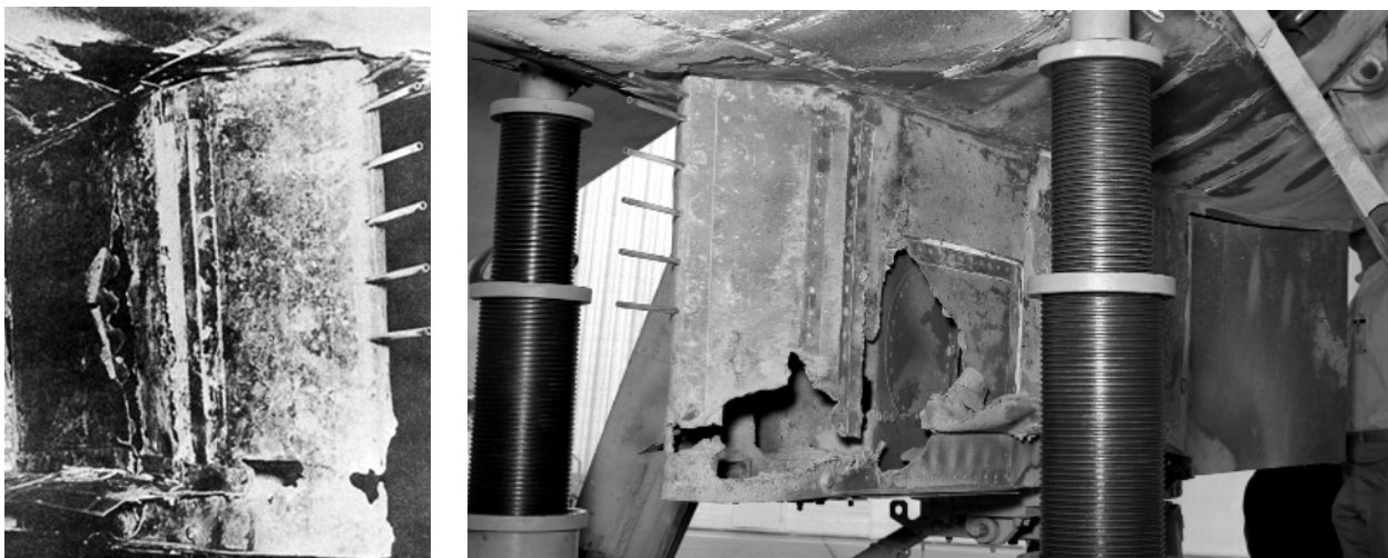
Figure 2-5. Damaged X-15-2 pylon from Mach 6.7 shock interference heating (images reproduced from a NASA report [9]).
