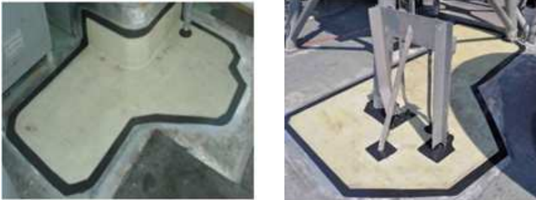
(a) Composite patch in machinery room.
