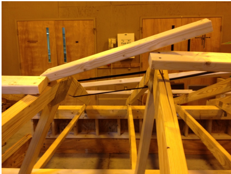
Figure 3-20: Withdrawal from the trusses
