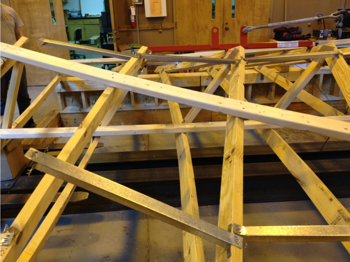
Figure 3-34: Spreader bar and engineered steel bracing failure
