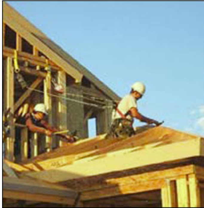
Figure 1-5: Residential construction worker using a PFAS (OSHA, 2010)
