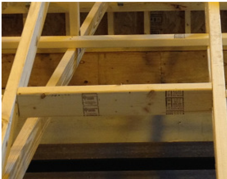
Figure 2-3: Wood bracing installed in-between trusses
