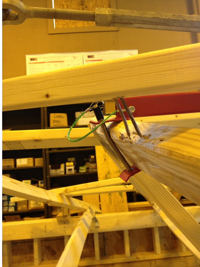
Figure 3-32: Failure in the diagonal bracing and anchor
