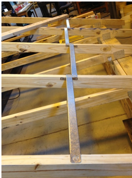
Figure 3-10: Engineered steel bracing installation
