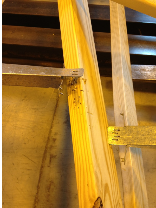
Figure 3-35: Failure in the engineered steel bracing
