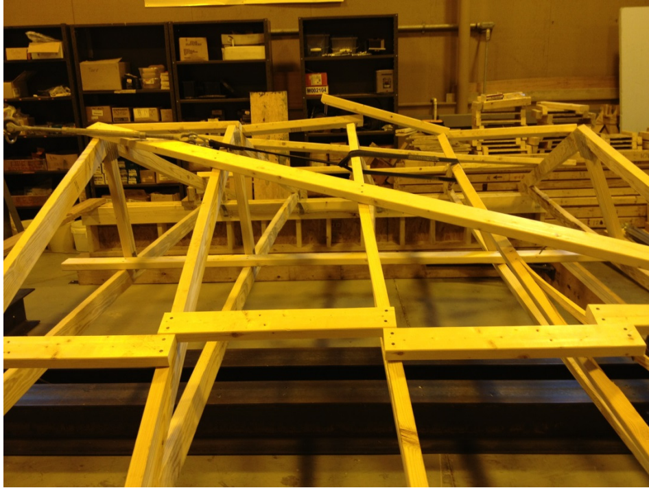
Figure 3-19: Failure in the on-top wood bracing & diagonal bracing
