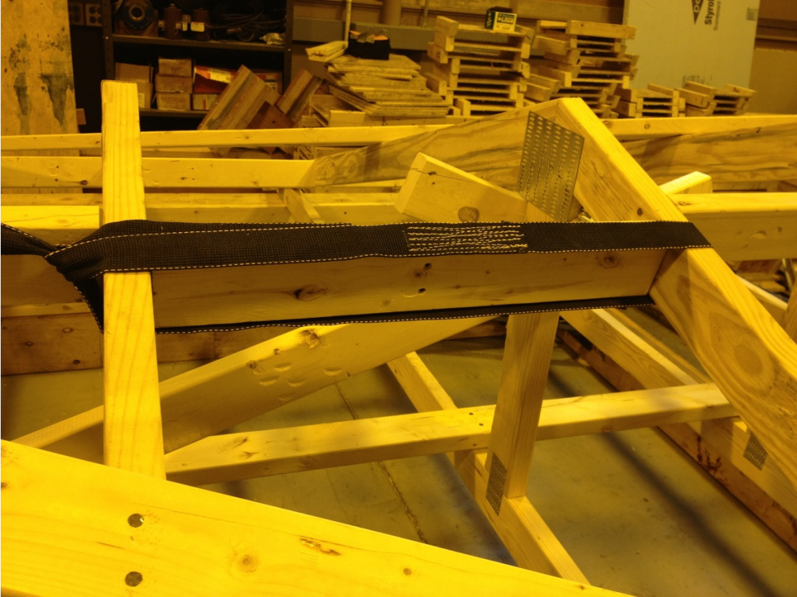
Figure 3-38: In-between bracing placed on the same side as the anchor
