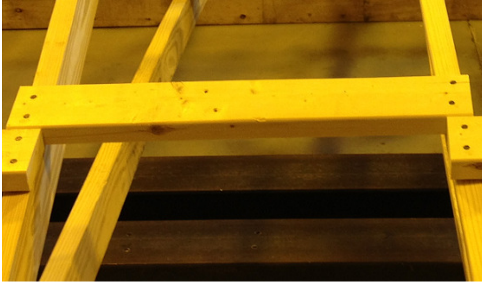
Figure 2-2: Wood bracing installed on-top of trusses
