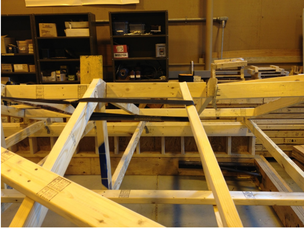
Figure 3-16: Cross-arm strap and in-between wood bracing
