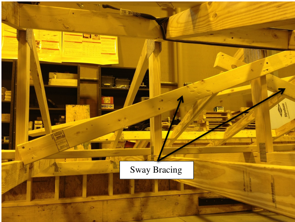
Figure 2-12: Sway bracing attached to king posts of a truss system
