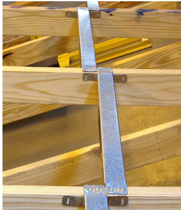
Figure 2-4: Engineered steel bracing installed in-between the trusses
