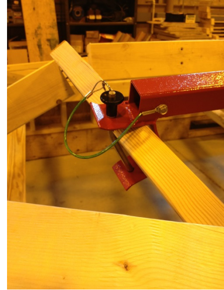
Figure 3-29: Failure in spreader bar
