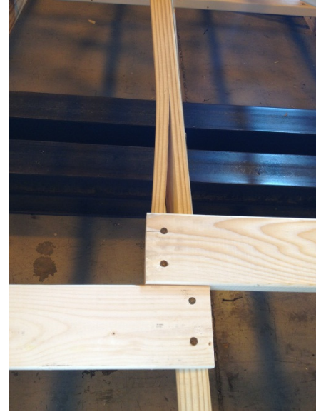
Figure 3-7: Truss splitting with PFA
