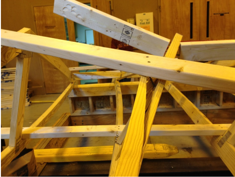
Figure 3-28: Failure in bracing and trusses
