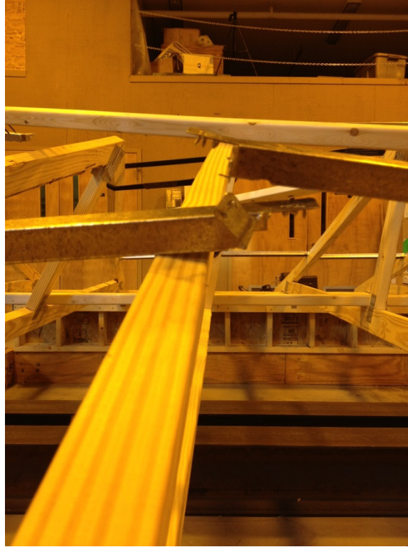
Figure 3-24: Failure in the engineered steel bracing
