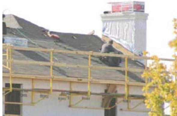
Figure 1-3: Worker utilizing a guardrail system while working on a roof (OSHA, 2010)
