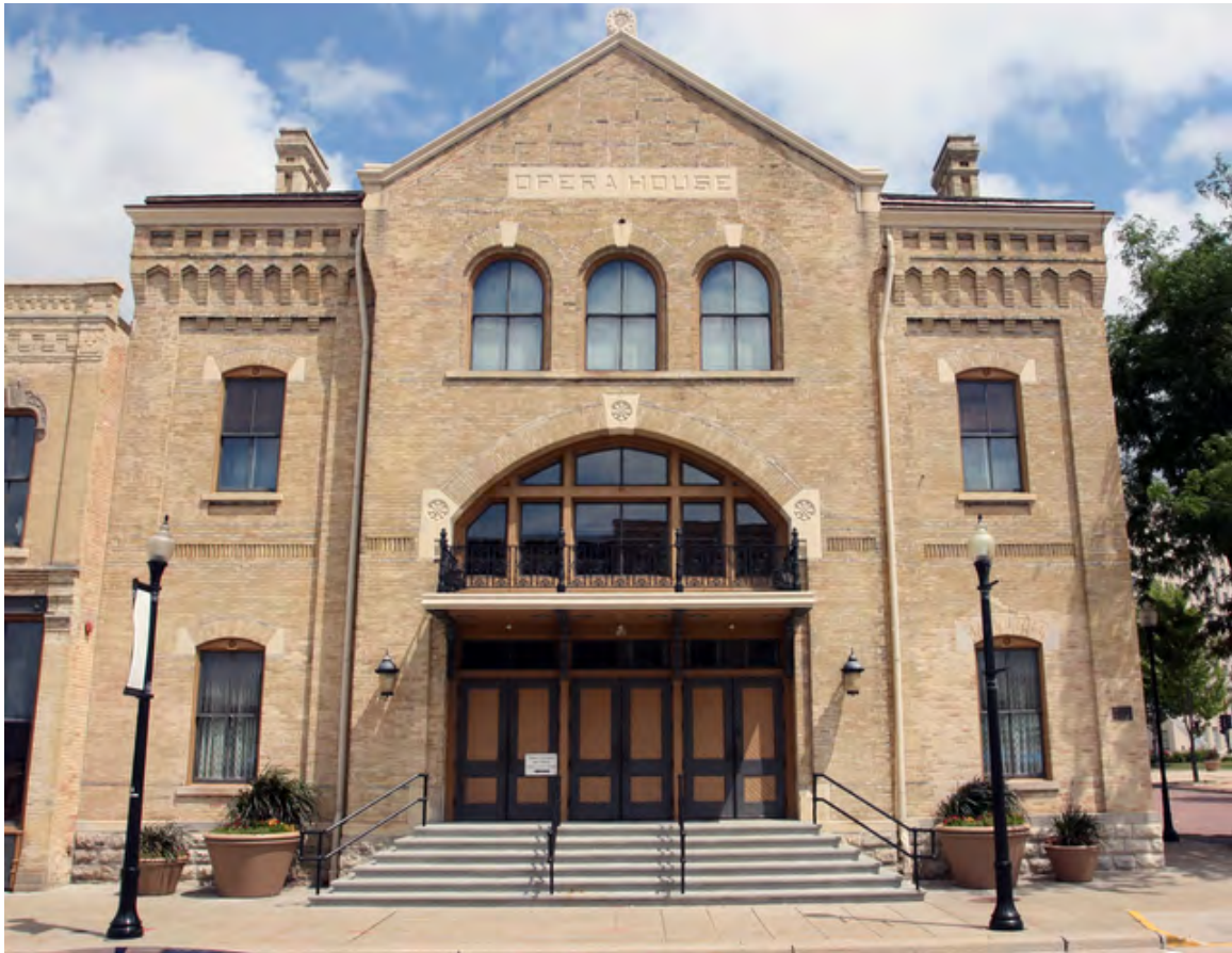
Image 13: Photograph of the main entrance of the renovated Grand Opera House
