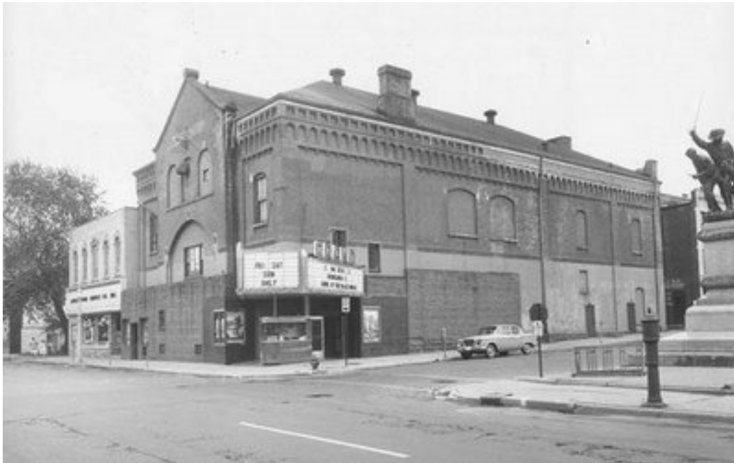
Image 12: Photograph of the dilapidated opera house with the entrance moved to the corner of the building
