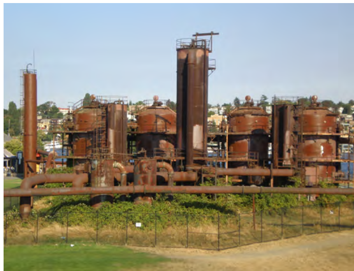
Image 18: View of the isolated cooling towers at Gas Works Park
