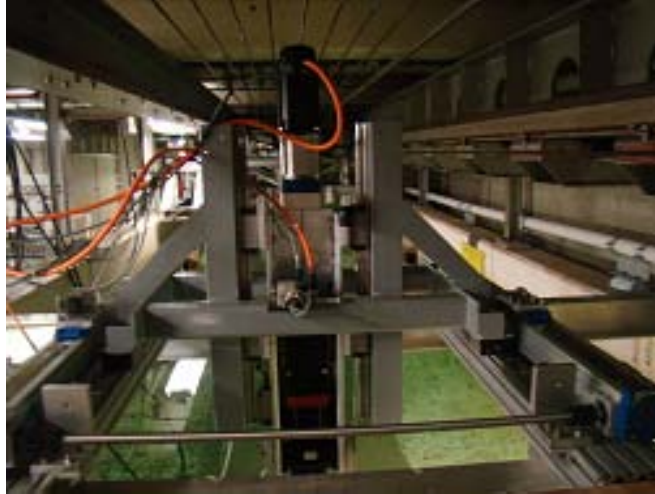
Figure C-16. Installation of the 3DoF motion mechanism in the NSWCCD 140 ft basin
