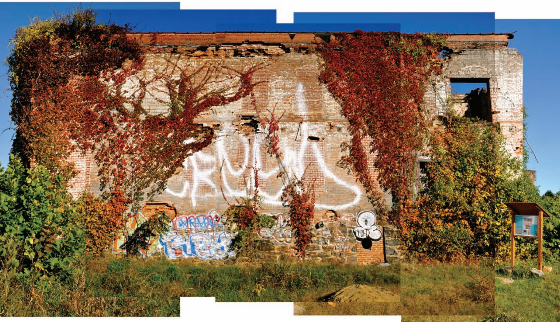
(Above) Photograph of the Asheville Cotton Mill's southern wall which has been taken over by the natural vegetation on the land. (Right, clockwise from top) The present day ruin and historic footprint of the Asheville Cotton Mill; the recently constructed Cotton Mill labyrinth; a sketch of the front elevation of the ruin.
