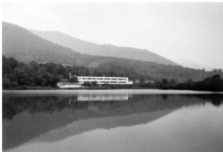
The Studies Building on Lake Eden. This building was designed by A. Lawrence Kocher from the Architectural Record and was constructed by students and faculty.
