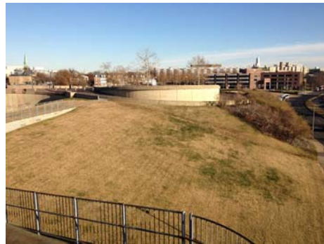
Banneker Overlook from 12th Street overpass
