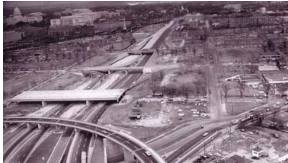
Southwest Freeway under Construction (Pg. 65)
