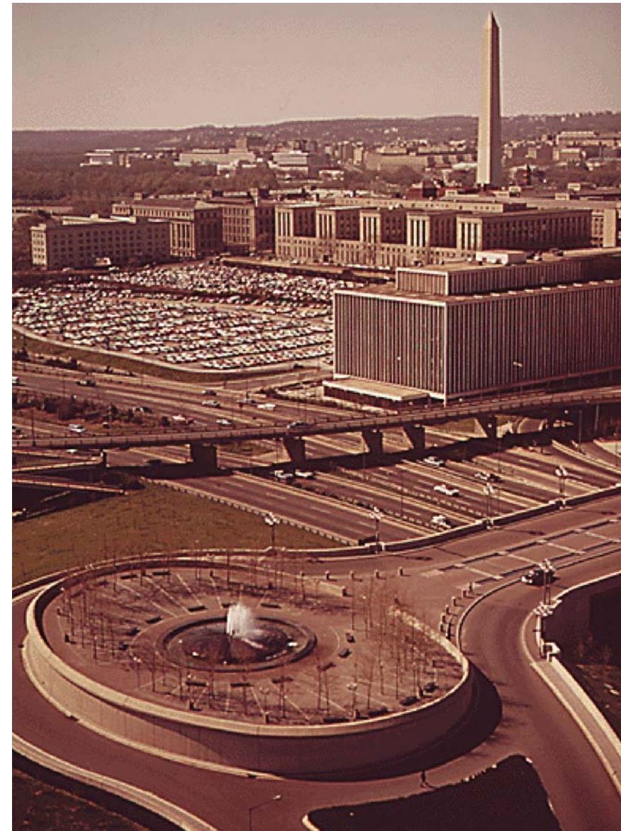
Banneker Overlook after Construction Completion, 1973 (Pg. 65)
