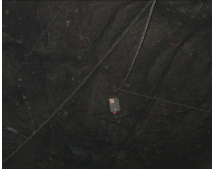
Figure 3.3: Methane Sensor Mounted Near Roof Outby Active Mining
