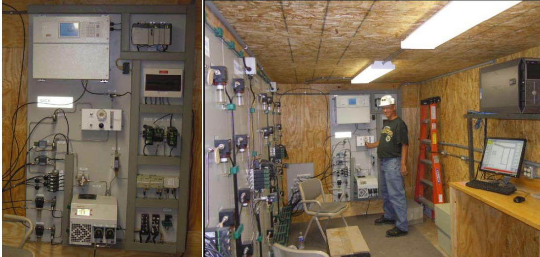
Figure 3.7: Analysis Unit Mounted on the Back Interior of the Trailer (Left) and Full View of Interior of Trailer (Right)
