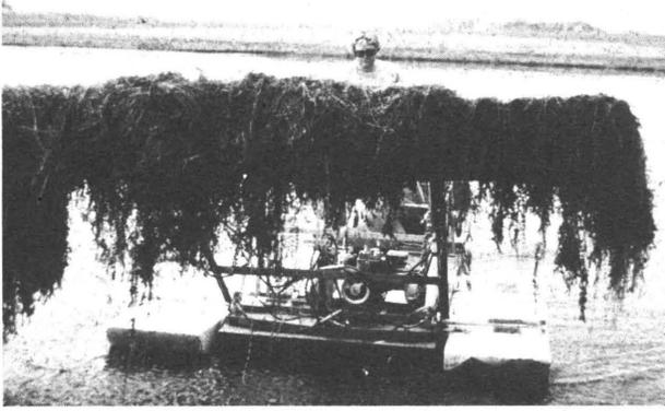
In shallow shoreline areas, weeds can be pulled by hand, cut by sickle, dug out with a hoe, and removed from the water with rakes or forks. In large ponds, a variety of commercial powered cutting machines are available. Some cutting blades can be mounted on the bow of a motor boat.
