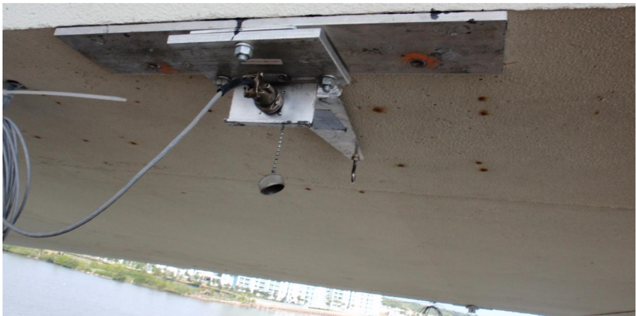
Figure 21 – Deflectometers on Bottom Slab of Seabreeze Bridge
