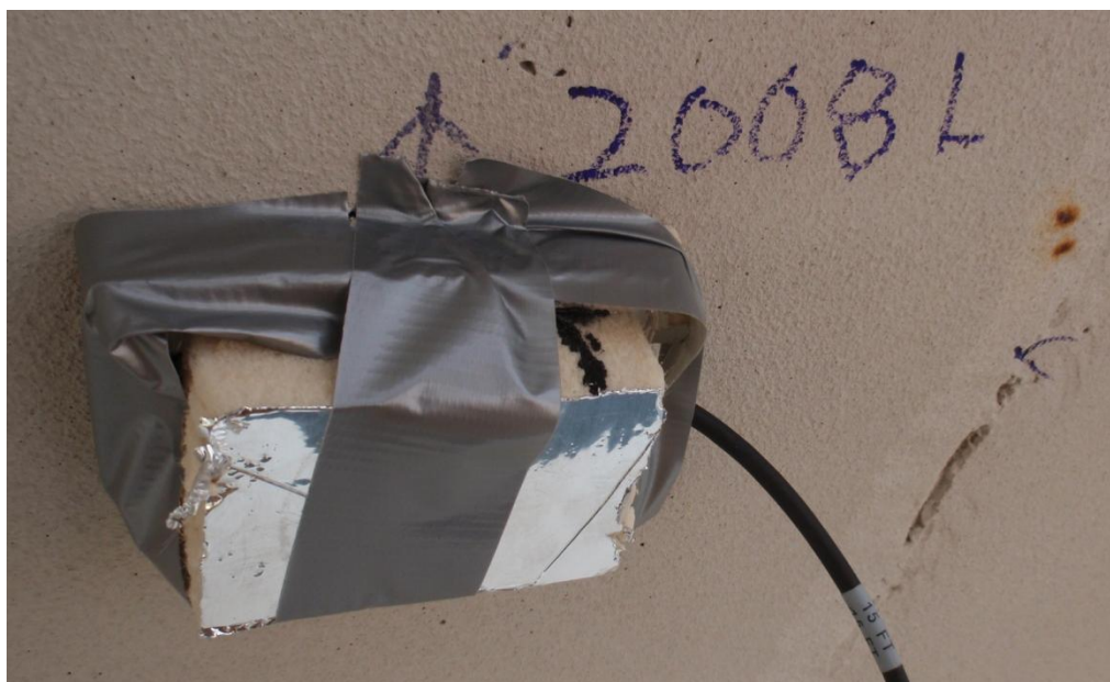
Figure 20 – Strain Transducer 2008 with Weather Protection
