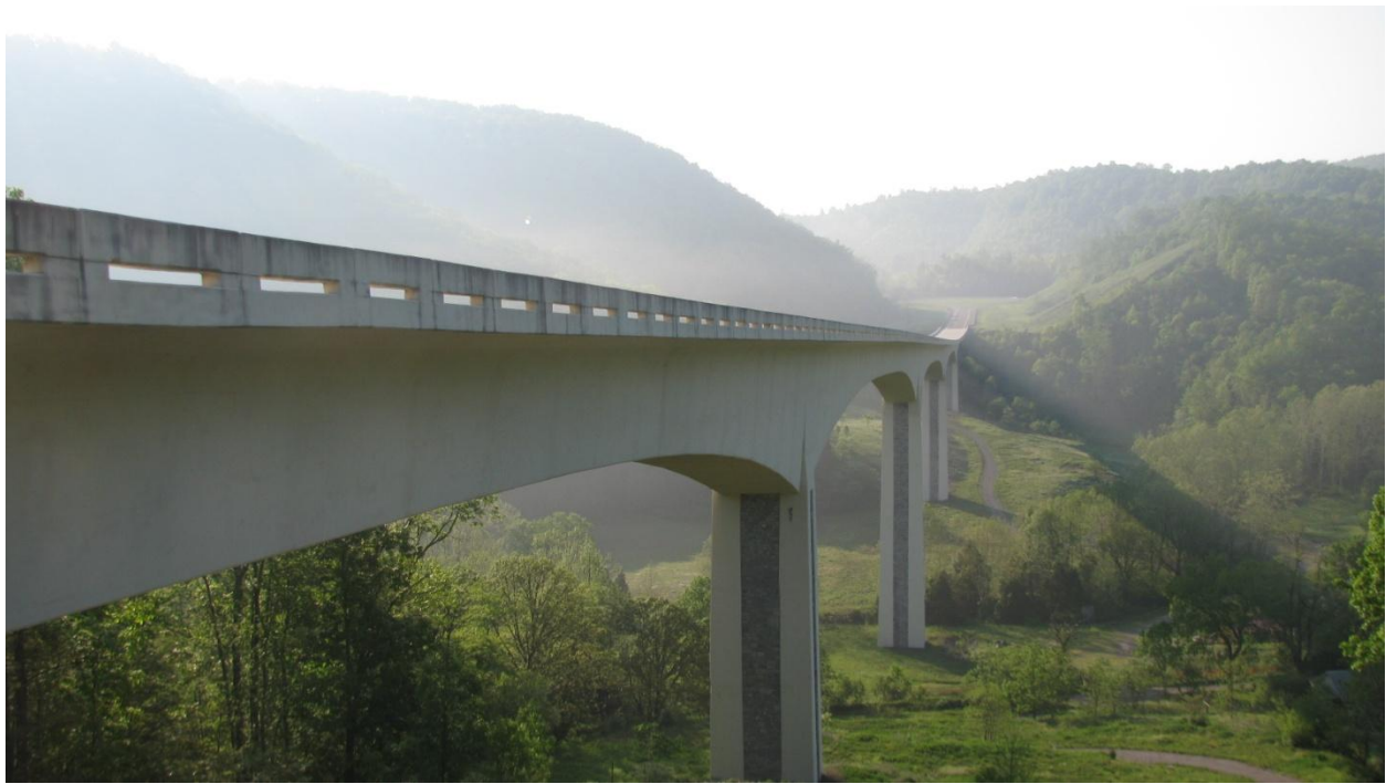
Figure 36 – Smart Road Bridge Spanning Ellet Valley near Blacksburg, VA
