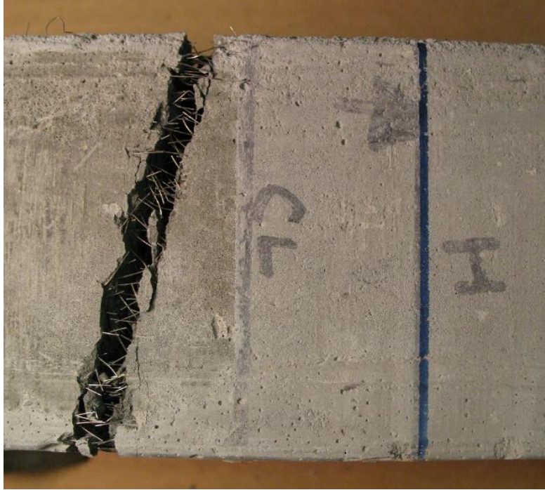
Figure 6-29: Failure surface of SP-D2 (bottom of web), where I is the intersection point of UHPC flow and CL is the center point of the rib.
