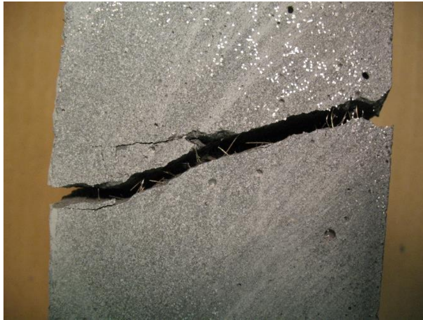
Figure 6-21: Failure crack of UD-A1 (top of web).
