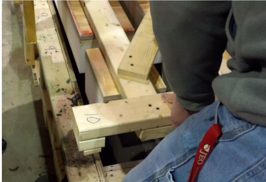
Figure 3-51: Foam attached to a frame was placed into DS-1 to create the ribs.
