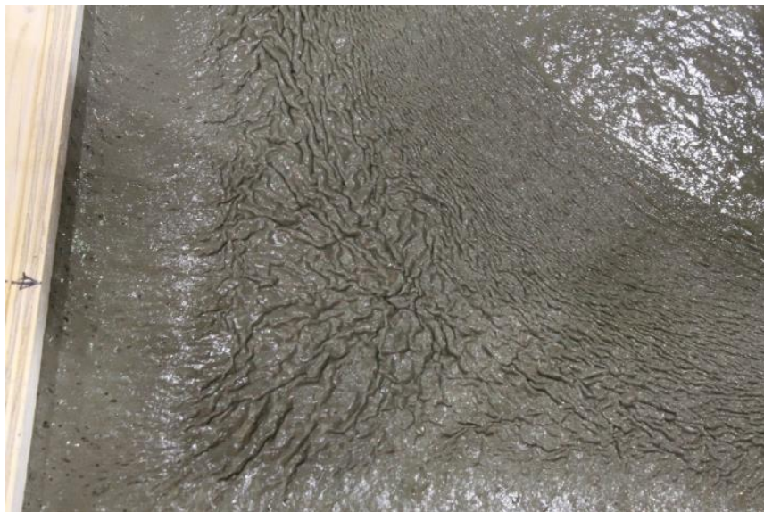
Figure 6-13: Exposed surface of UHPC during top-side up corner placement, scenario A (Photo by K. Halbe).
