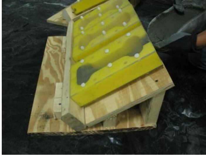
Figure 3-25: UHPC was placed at a 33.9° angle to control fiber orientation.
