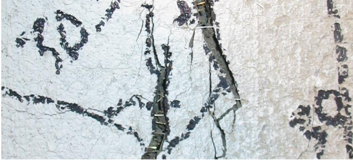
Figure 7-31: More dense fiber network on DIC side of beam displayed fiber bridging.
