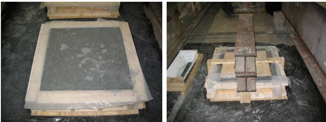
Figure 3-43: Exposed UHPC was covered with plastic sheeting to contain moisture.
