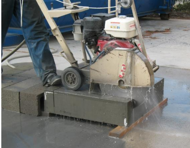
Figure 3-45: A walk-behind concrete saw cut the webs from the single cell units.
