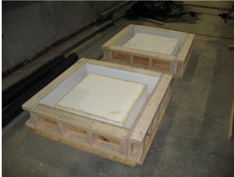
Figure 3-37: Single cell formwork containing foam for top-side up placements.
