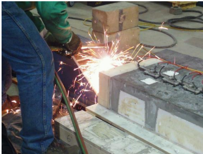
Figure 3-57: Prestressing steel was cut by heating strands using an acetylene torch.
