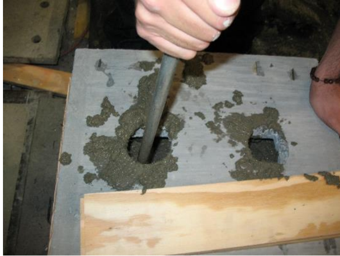
Figure 3-66: Grout-filled shear pockets were consolidated using a tamping rod.
