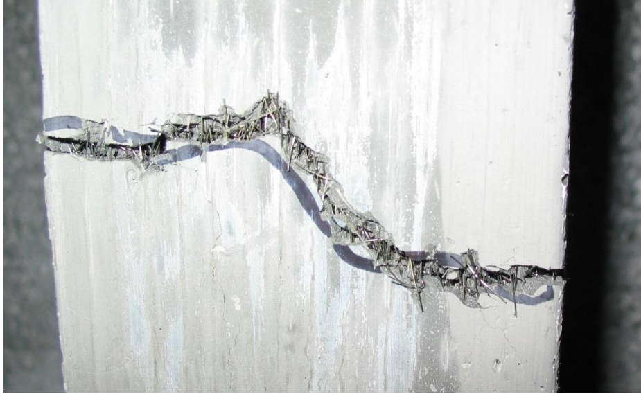
Figure 7-33: Underside of the web showed a high concentration of fibers bridging the dominant flexure crack.
