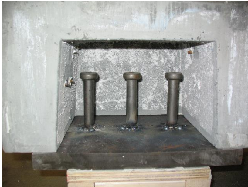
Figure 3-64: The plates and studs were aligned with the deck section shear pockets.
