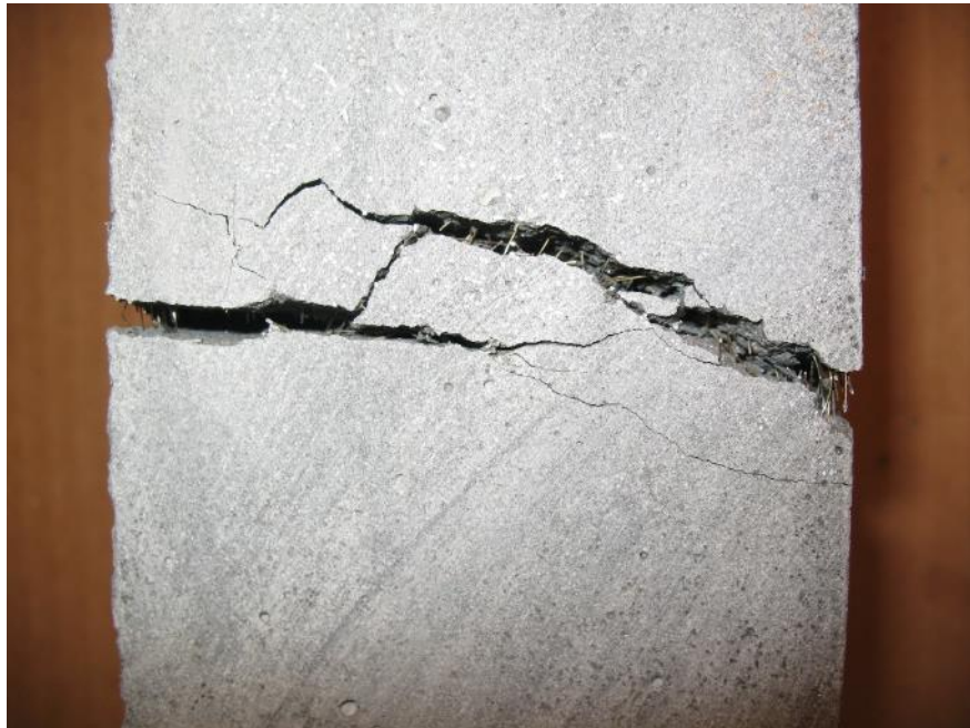
Figure 6-23: Failure crack of UD-C1 (top of web).
