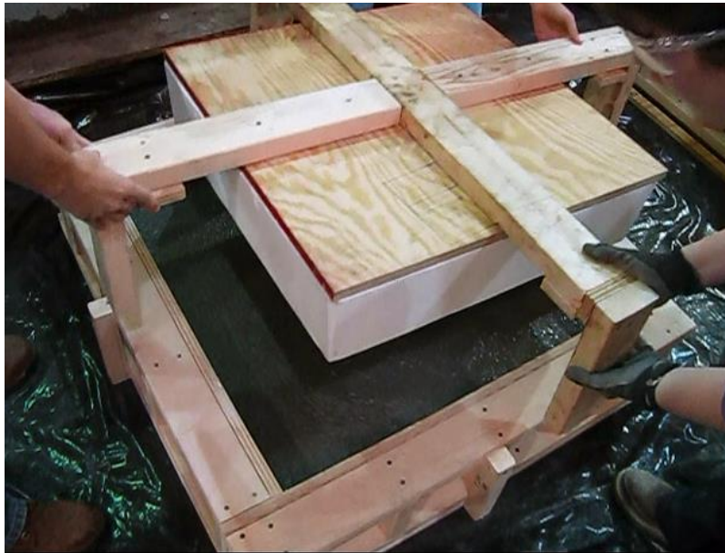
Figure 3-41: The frame was inserted into the form to create the ribs (Photo by K. Halbe).
