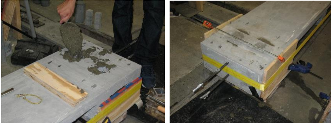
Figure 3-65: The top plywood form was added after UHPC filled the shear pocket.
