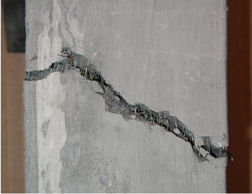
Figure 6-26: Failure crack of SP-C2 (bottom of web).
