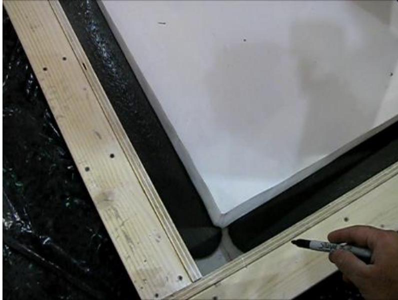
Figure 6-9: UHPC intersected near the opposite corner of flow entrance for placement scenario A (Photo by K. Halbe).
