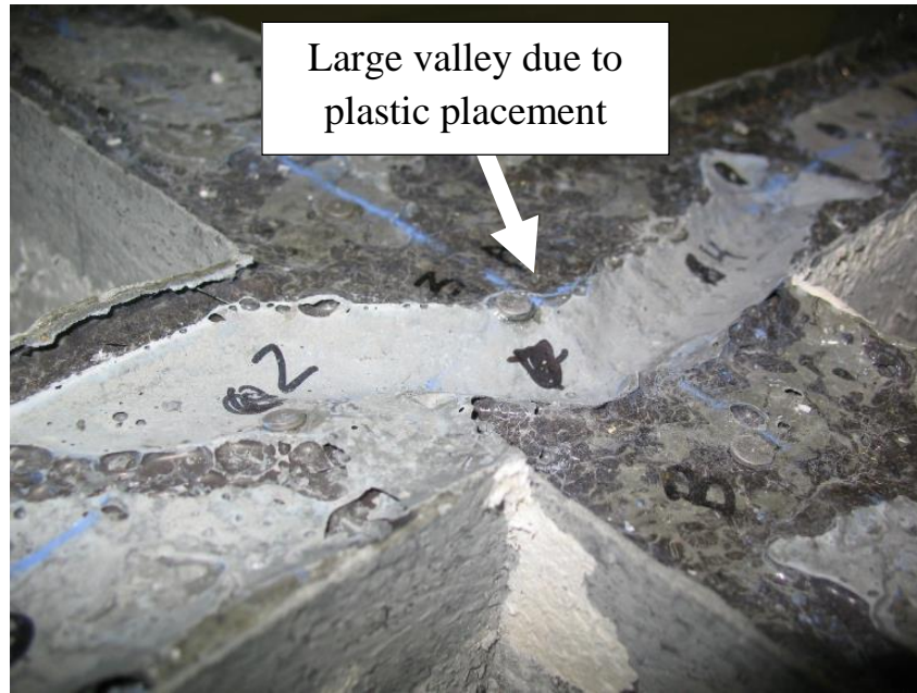
Figure 7-2: Surface abnormalities occurred due to faulty plastic placement.
