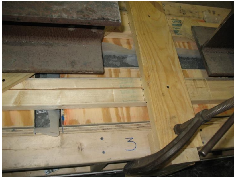
Figure 7-1: Some difficulties occurred in placing plastic on exposed UHPC because of the frame.
