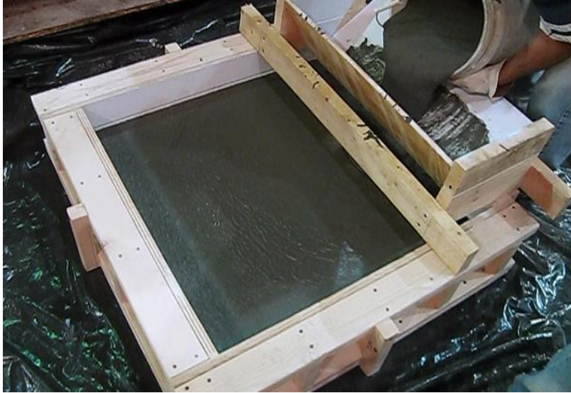
Figure 3-40: UHPC was placed in an open form for the upside down placement (Photo by K. Halbe).
