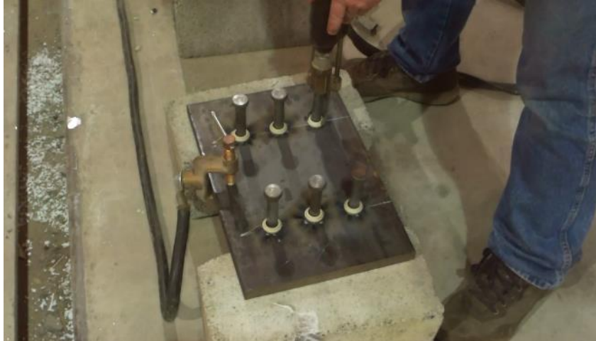
Figure 3-63: Shear studs were welded to a 1 in. thick steel plate (Photo by M. Maguire).
