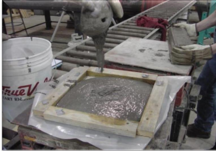
Figure 3-11: Placement of small UHPC panels.
