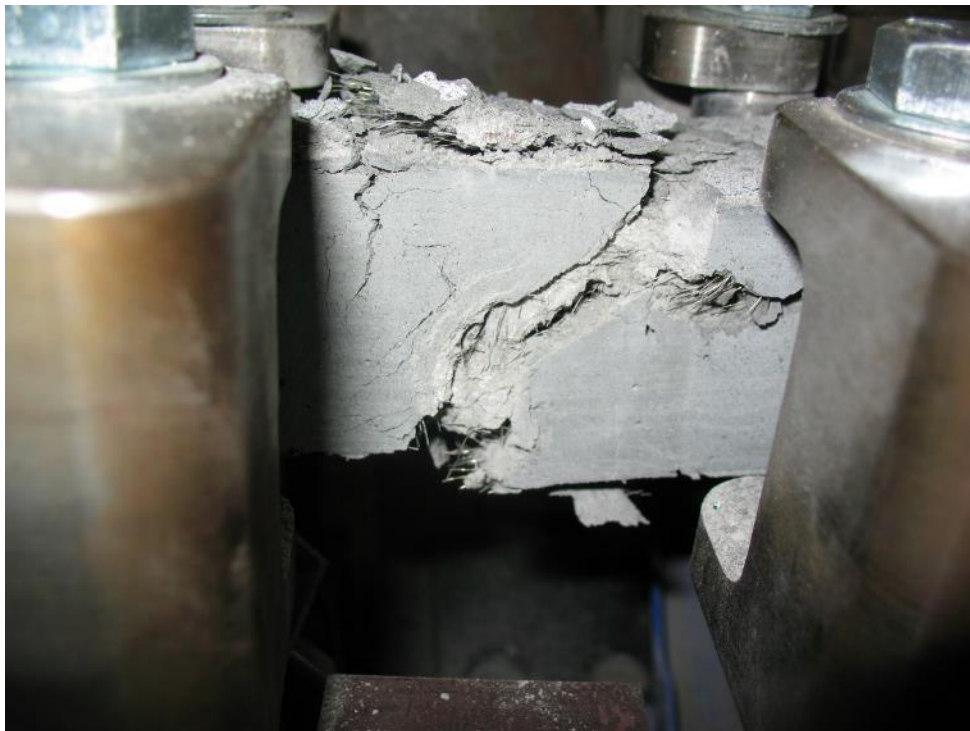
Figure 5-21: Inclined cracks were common among UT-I failures (PC-2).
