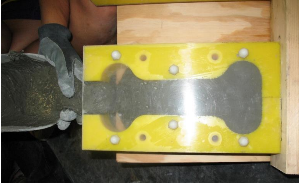
Figure 5-3: UHPC was funneled manually to place into forms.
