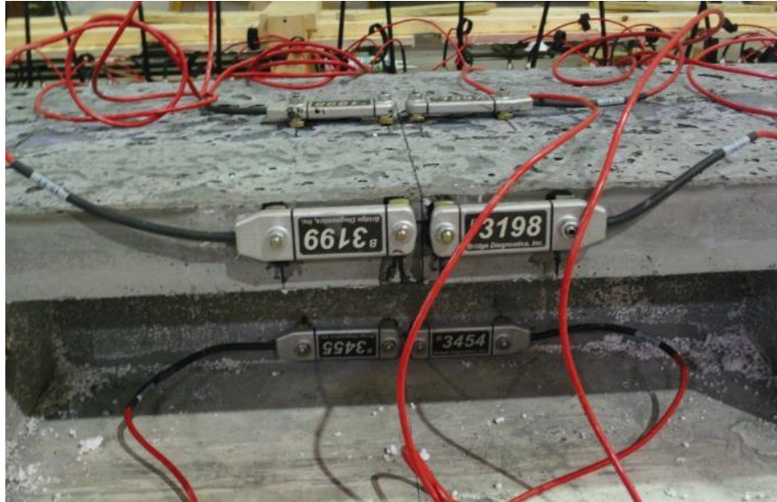
Figure 3-62: BDI gages were placed at the middle of DS-2 to determine the effective prestressing force.
