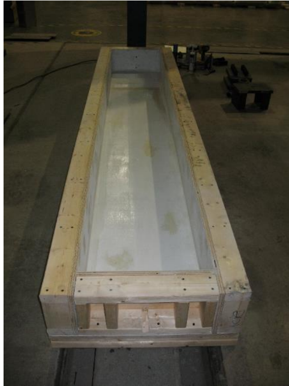
Figure 3-48: Formwork was constructed using 2x4 lumber and 0.75 in. plywood.
