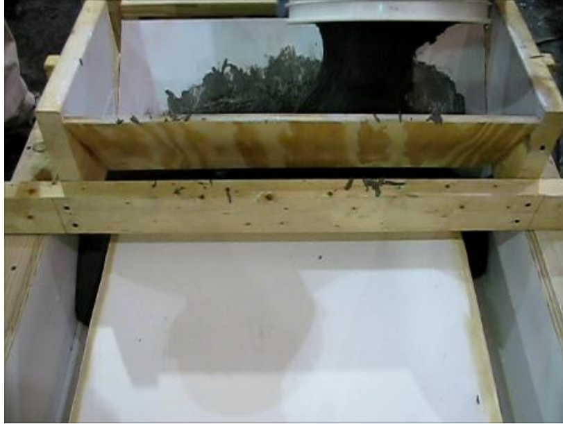
Figure 3-38: UHPC was inserted into one rib for the side placement method (Photo by K. Halbe).
