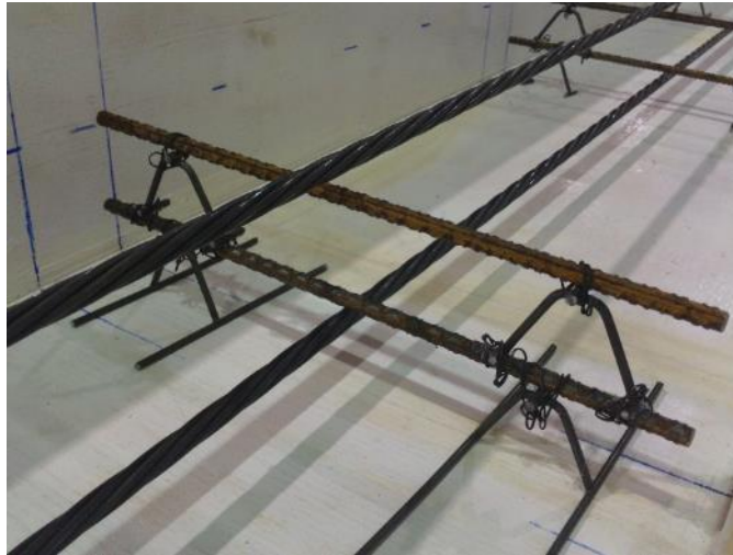
Figure 3-49: Reinforcing bars were placed using chairs in DS-1.
