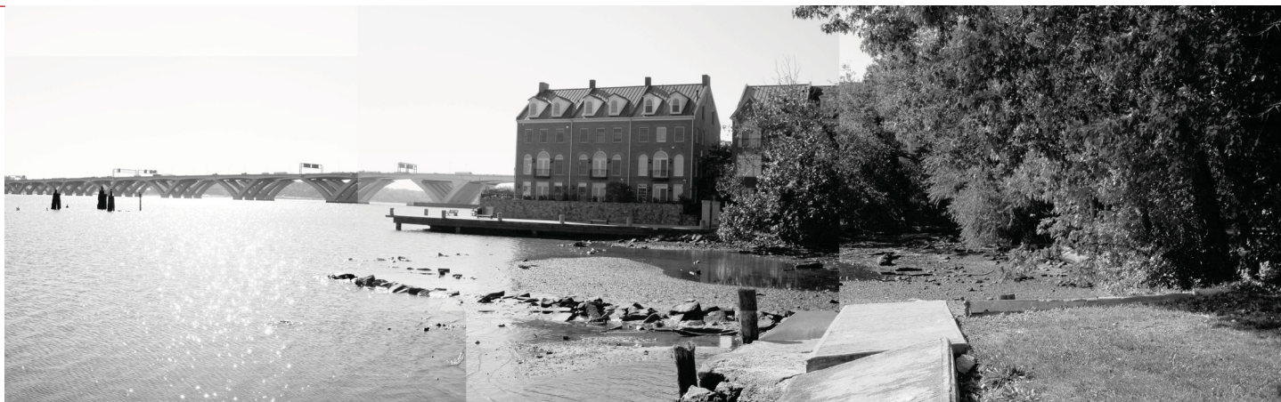
view of the waterfront looking south
