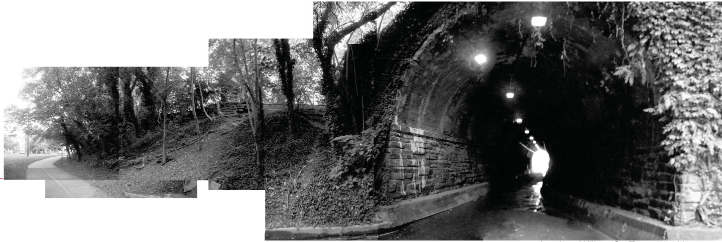
view into Wilkes St. Tunnel looking west
