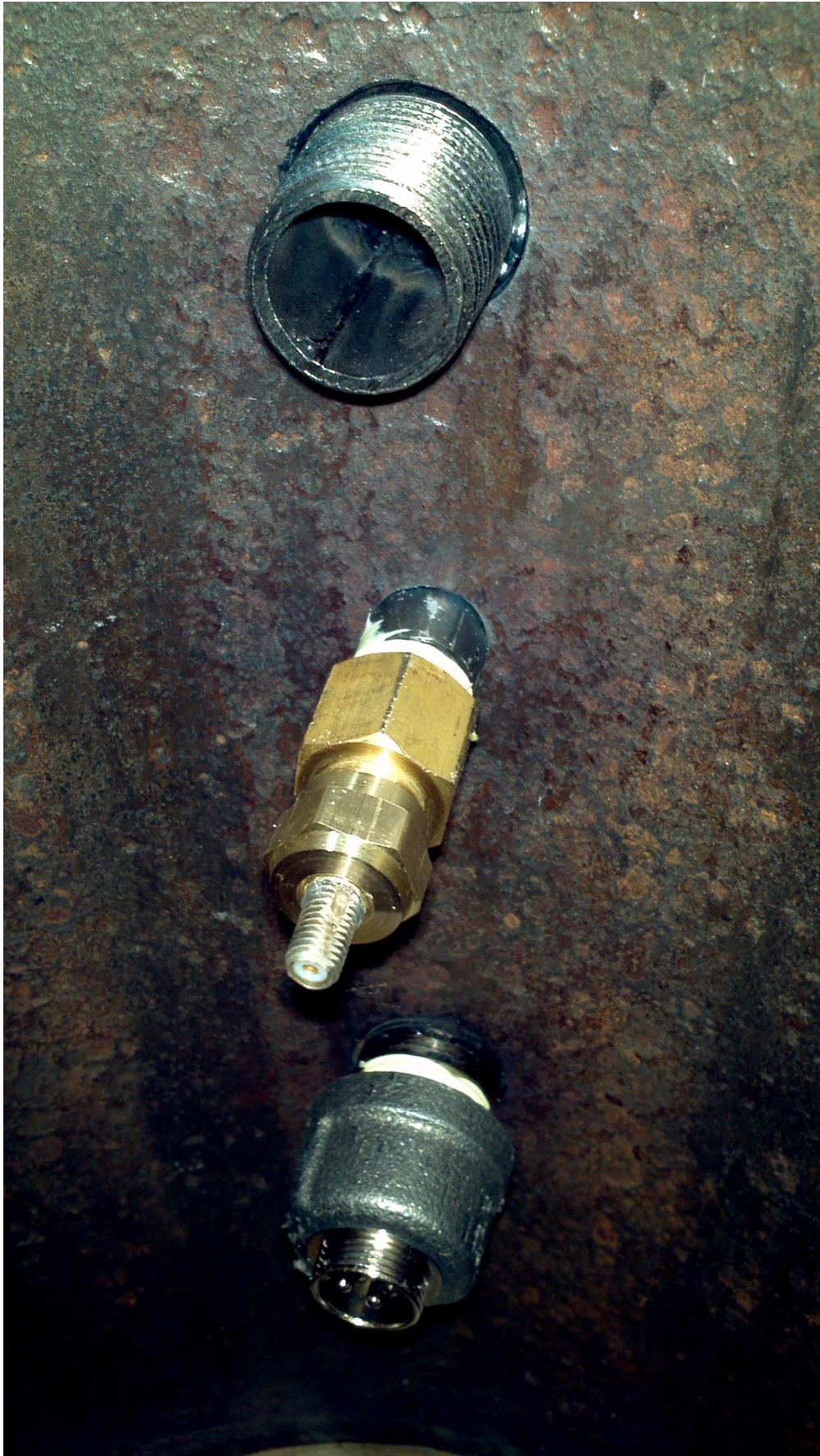
FIGURE 39. Pressure and Instrumentation Ports as Viewed from Inside the Cavity
