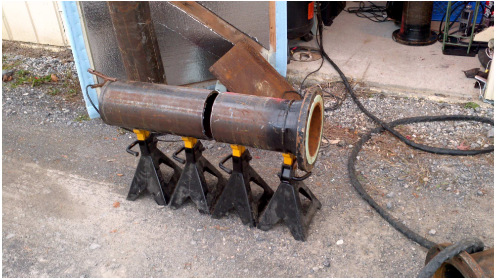
FIGURE 34. Original 8 in Diameter ANSI B36 Steam Pipes
