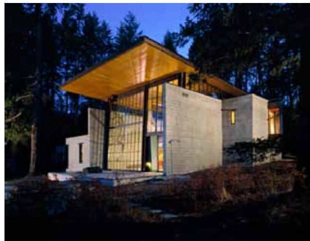
(Below) Chicken Point Cabin Exterior (Right) Chicken Point Cabin Stair
