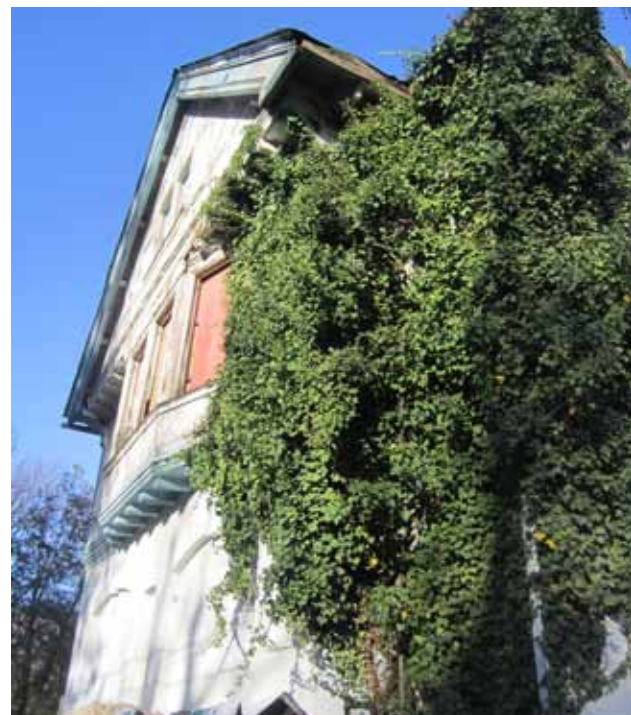
(Top) Truss connection (Middle) Stair addition (Bottom) Front facade
