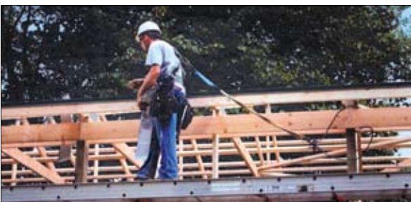
The research project will develop a more effective Fall Arrest System — a set of equipment used to prevent construction workers from falling while they perform their daily tasks.
