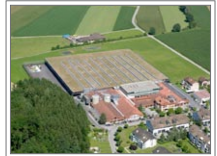
Figure 2: Baumgartner windows' new manufacturing facility (source: Baumgartner Fenster).
