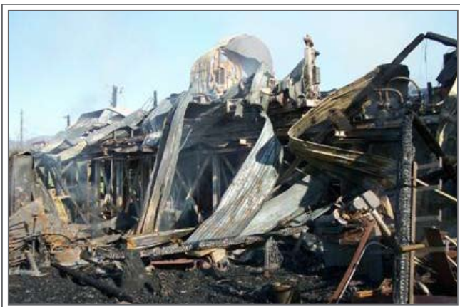
Band saw and carriage center, shop and saw file room left
