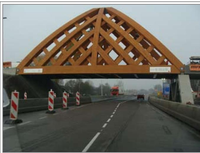
When designing their masterpiece, OAK Architects specified Accoya® wood because of its many benefits, including high strength to weight ratio, enhanced durability and dimensional stability, non-toxicity and aesthetics. The wood used in the bridge’s dramatic design not only makes it look impressive but performs also the important function of bearing the traffic load.
