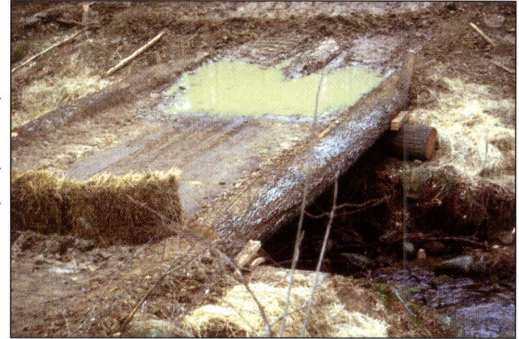
Bridges can be long-term road structures or simply a temporary structure for crossing a stream.
