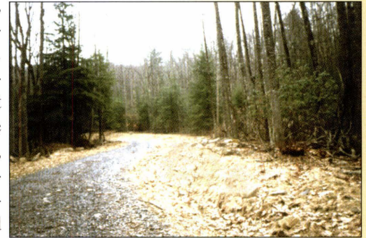
A daylighted road will receive enough sunlight to dry quickly.
