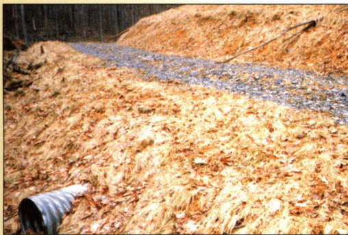
Slightly graded roads are more desirable than steep roads.
