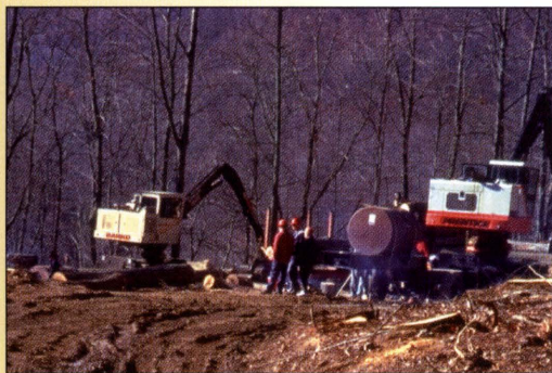
Proper location is a key in preventing erosion from a log landing.
