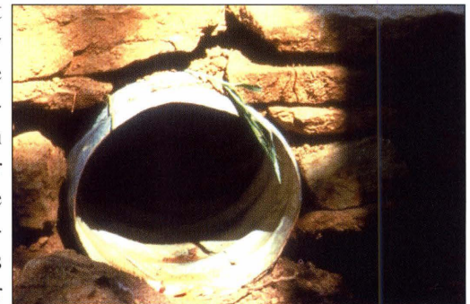
Culverts are commonly used in road construction.
