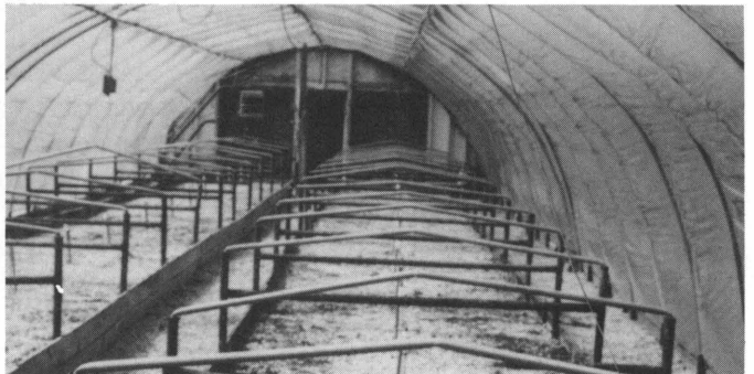
Quonset plastic greenhouse with inside benches covered for plant propagation. A house-within-a-house construction. Heat is provided by hot water pipes under the benches. This arrangement requires minimal heating. (Roadview Farm Nursery, Gloucester, VA)
